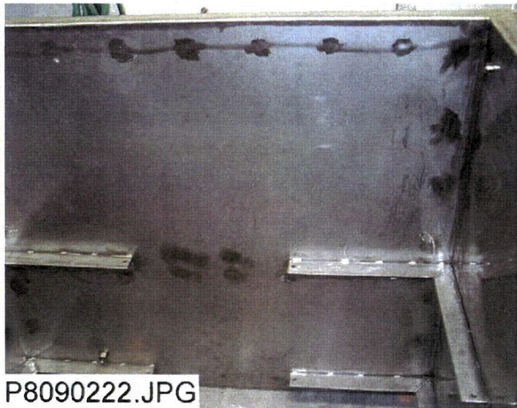
Figure 6. The top and bottom angle irons for supporting coupon racks in the upper section of the ICET tank.
