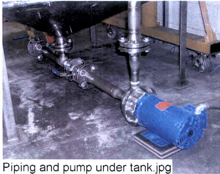
Figure 12. Circulation pump for the ICET system.
