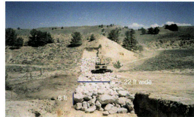
Placing Rock in Scour Apron (22 ft x 6 ft)
