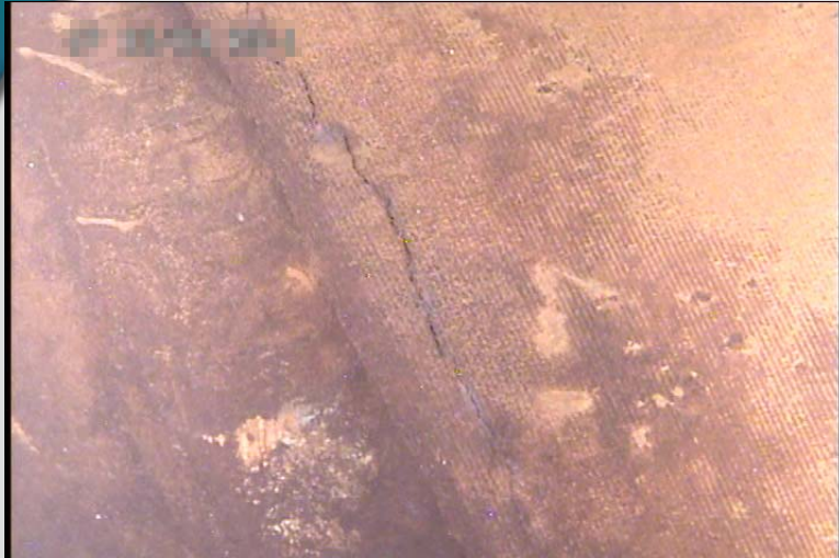
Definite Cracks
