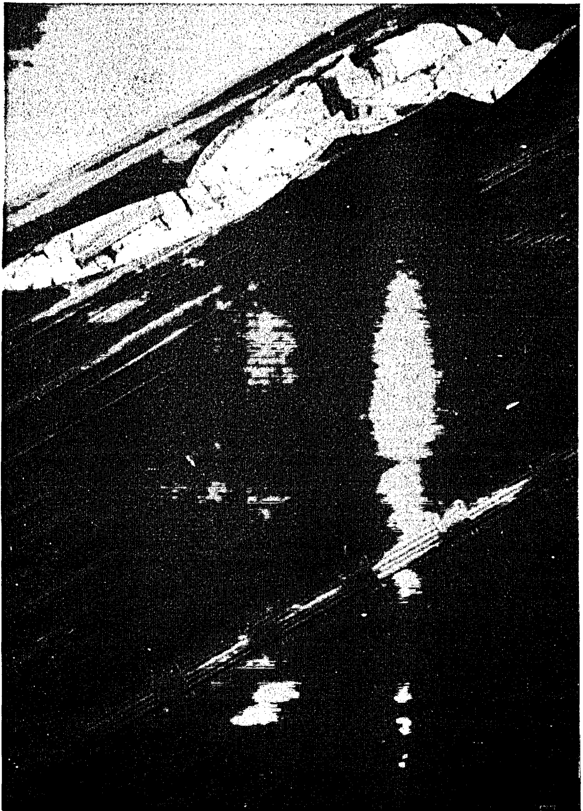
Figure 5. Close-up view of cracked region in the LP-FP-2 shroud.
