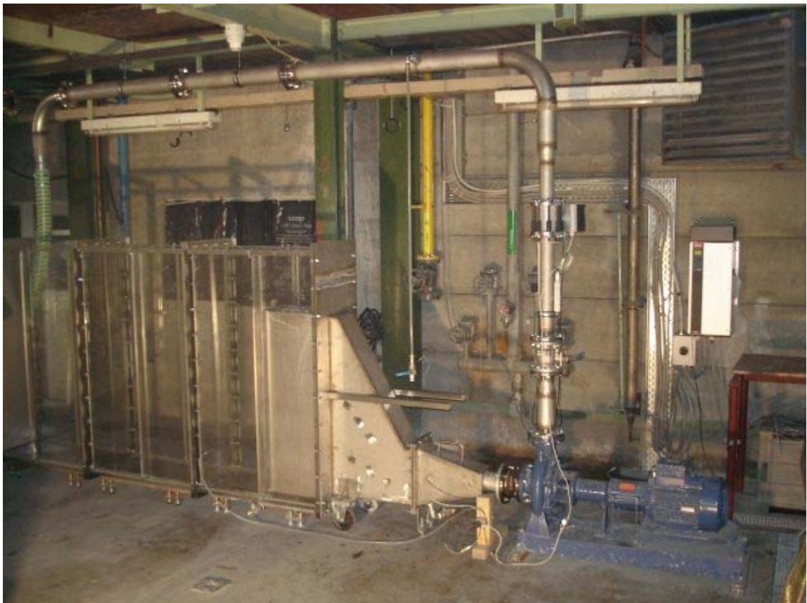
Picture 1: Multi Functional Test Loop (MFT-Loop)
