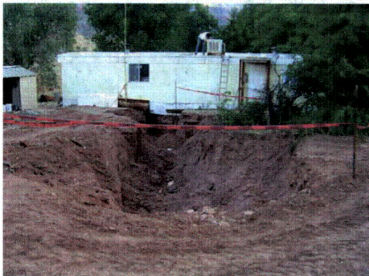
SU-2: Excavated trench next to resident trailer
