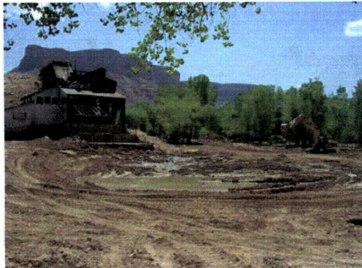
SU-4: Late excavations directly below mill building (groundwater level is where pond has formed)
