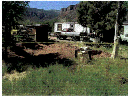
SU-3: Excavated pit near resident trailer
