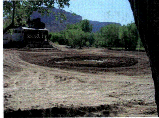
SU-4: Pond below mill after excavation and re-grading
