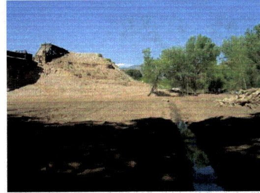
SU-5: New ditch constructed in Survey Unit 5 during re-grading
