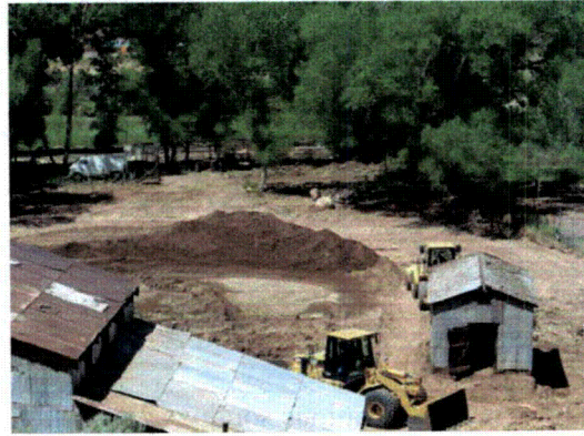
SU-4: Interim excavation and stockpiling of material in Survey Unit 4
