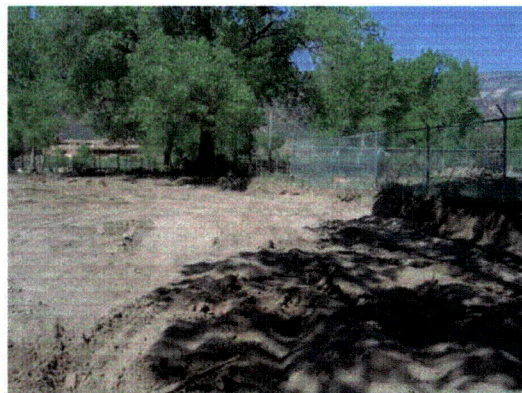
SU-4: Excavations next to CDOT fence
