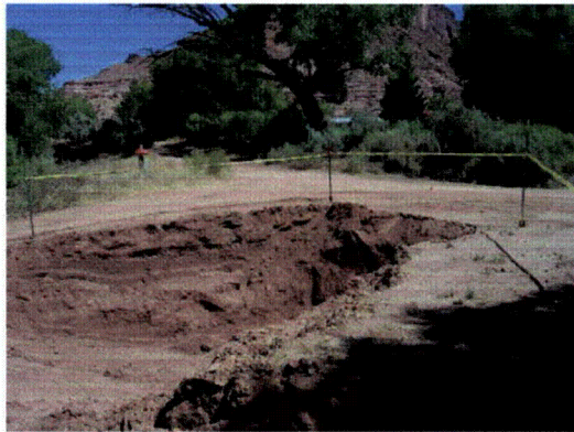
SU-3: Excavated pit near upper resident parking area
