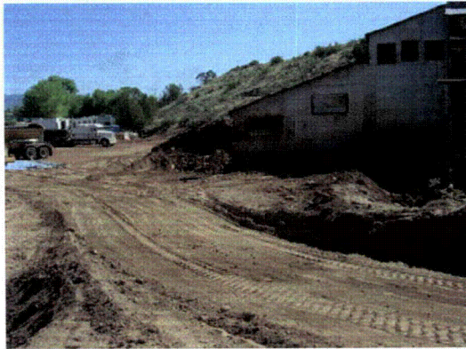
SU-4: Interim excavations near mill building and temporary haul road to load-out area
