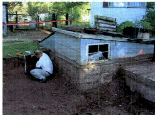
SU-2: Excavated pit at Willis root cellar trailer
