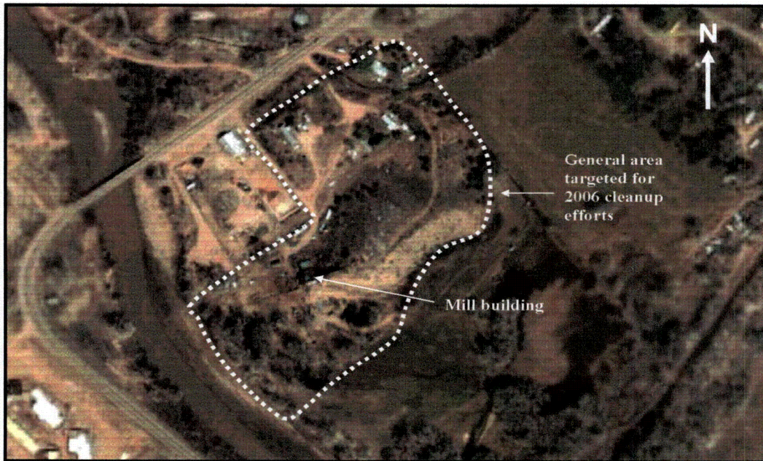
Figure 3. Aerial photo showing approximate boundary of areas targeted for potential excavation on mill site grounds during the 2006 cleanup project.
