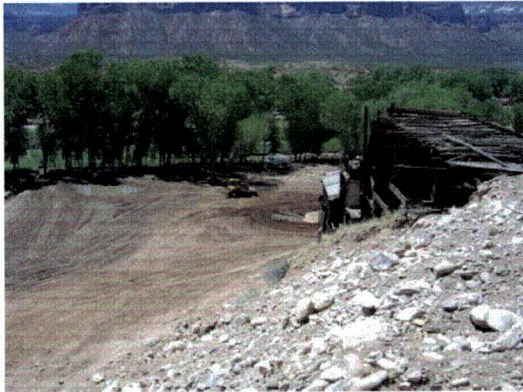
SU-5: Post-cleanup re-grading in Survey Unit 5
