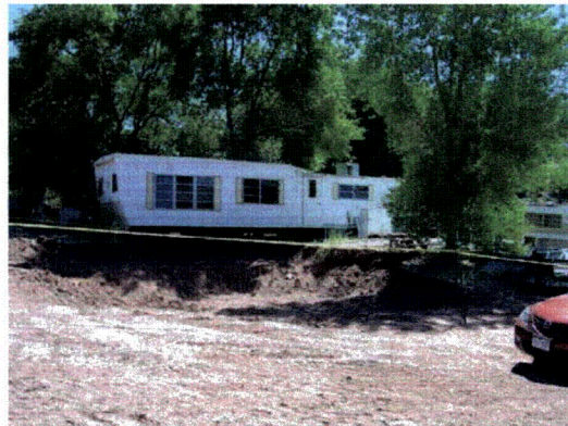
SU-3: Excavated pit near resident trailer
