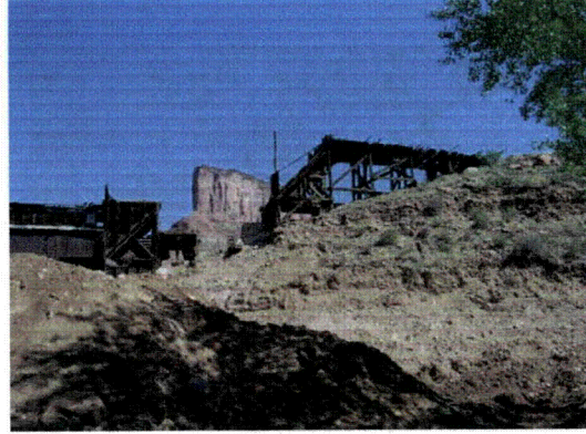
SU-5: Temporary stockpile of material south of mill building
