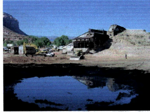
SU-5: Temporary pond formed southwest of mill building as excavations reached a little below groundwater table
