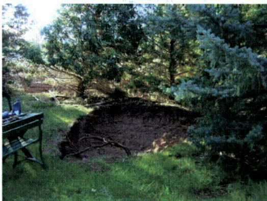
SU-2: Spot excavation pit in Willis yard
