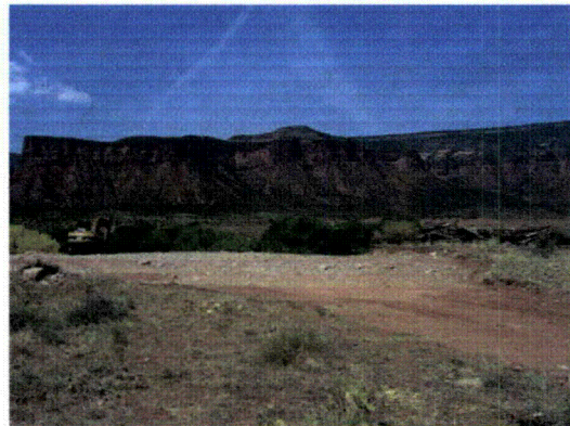
SU-1: Hill top above mill building after excavations
