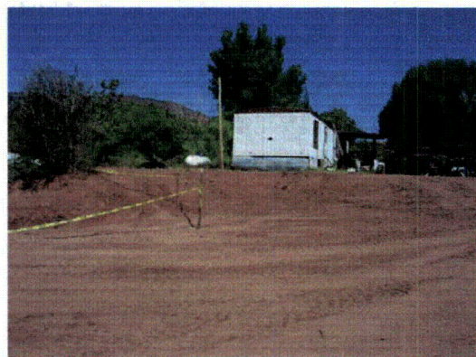
SU-3: General excavations near resident trailer
