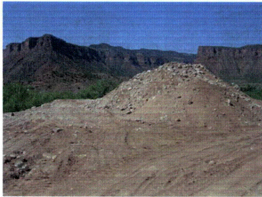
SU-1: Temporary stockpile of excavated material on hill top above mill building
