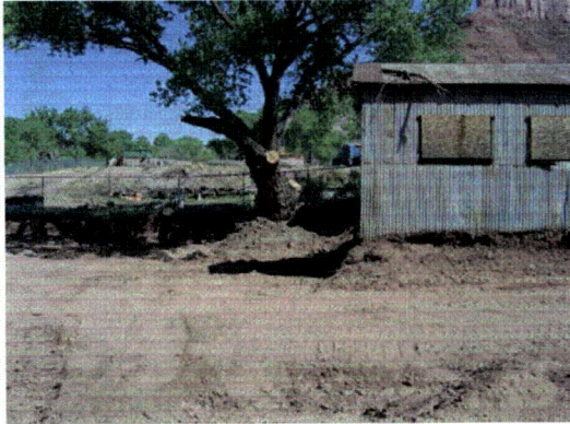
SU-4: Excavations next to CDOT fence (tree was later removed)
