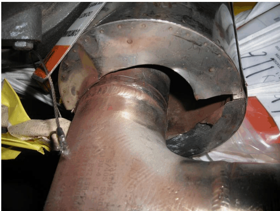
Figure 2: Insulation End-Cap to Pipe Interaction
