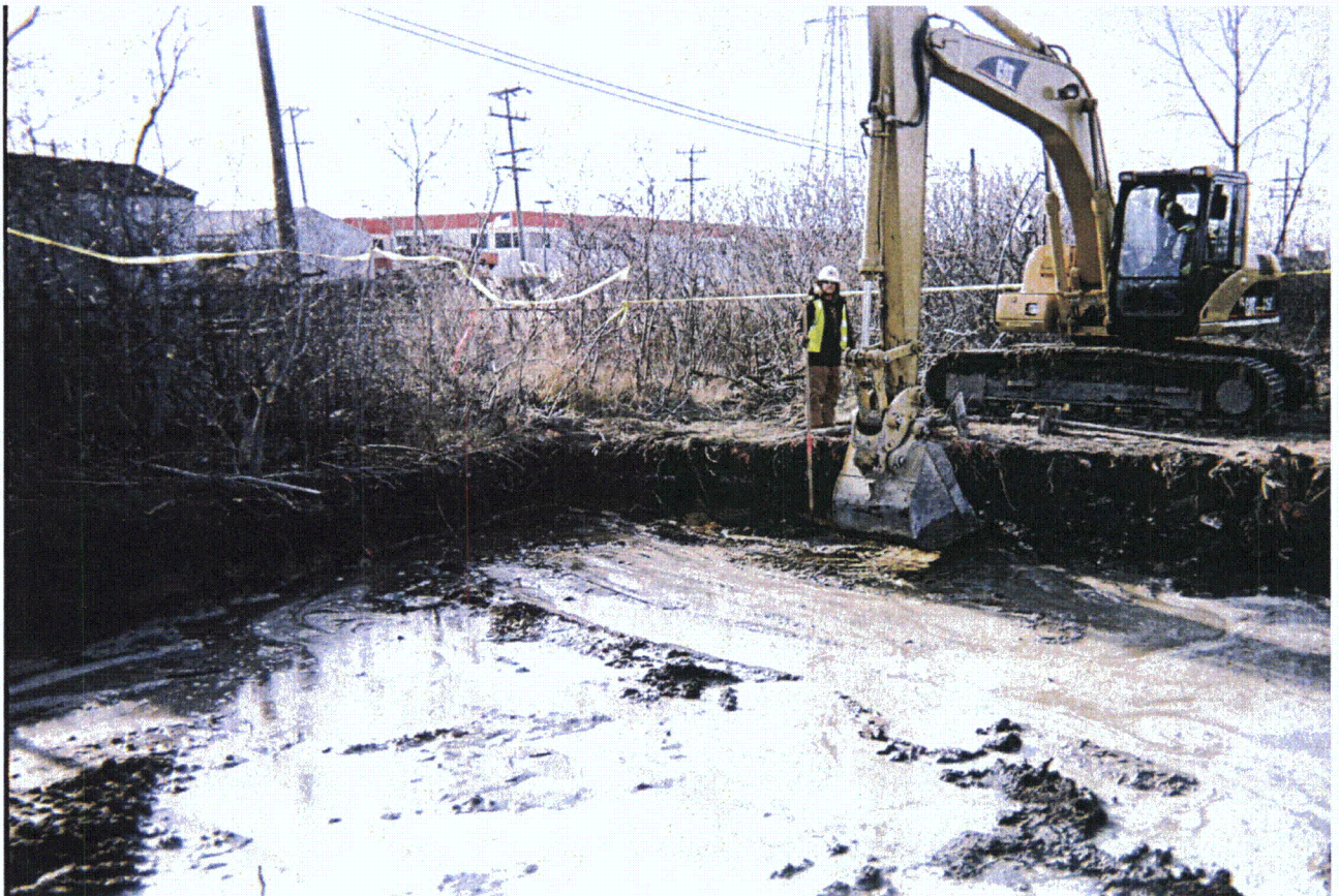
Photo 6 - Measuring depth of excavated grid.
