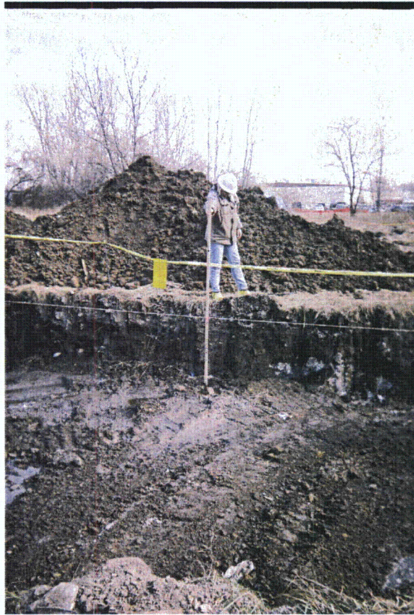
Photo 5 - Measuring depth of excavated grid.
