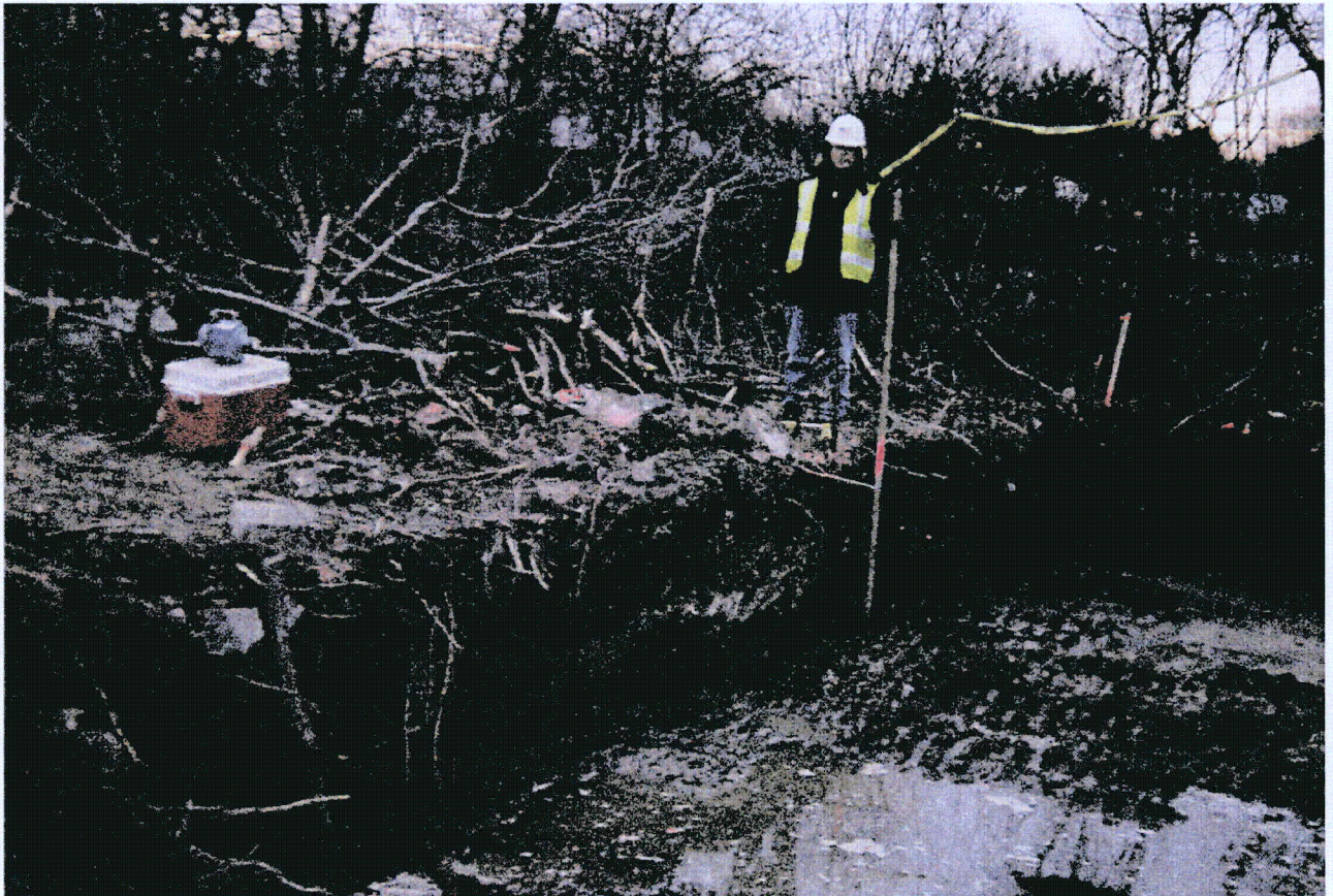
Photo 7 - Measuring depth of excavated grid.
