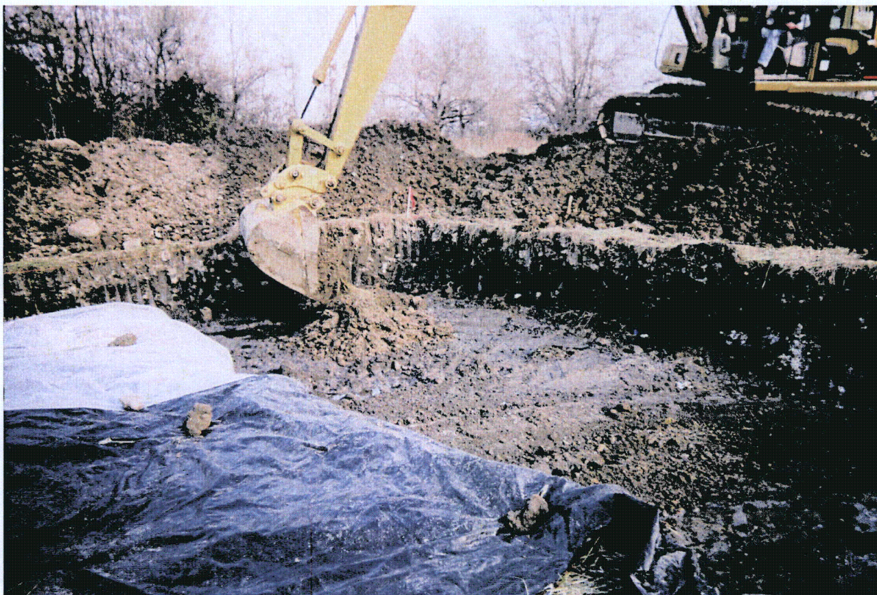
Photo 10 - Backfilling of excavated grids with clean fill.
