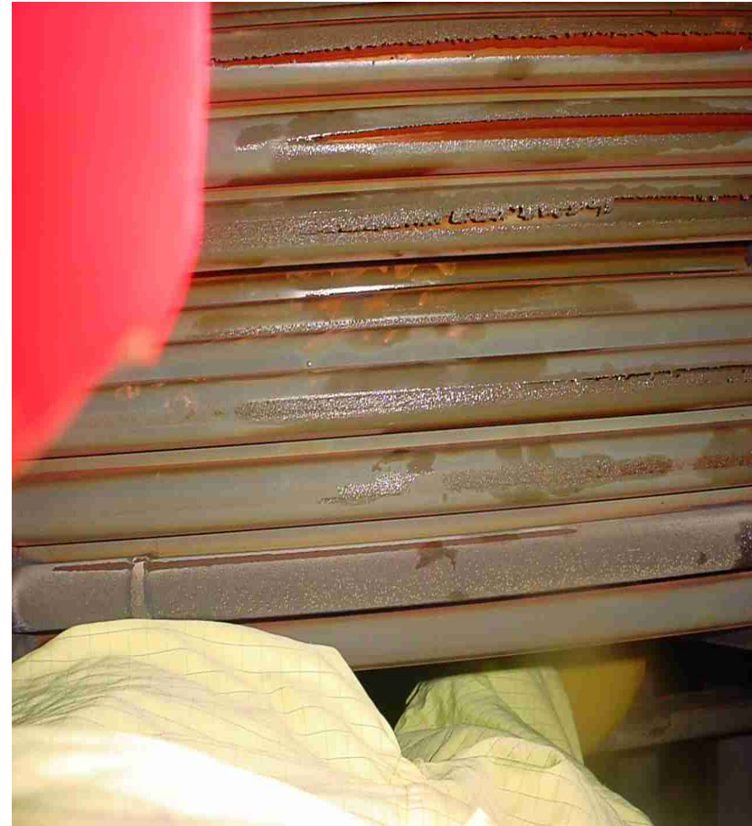
U2 Condenser South Side Eroded Tubes 06/08/2006
