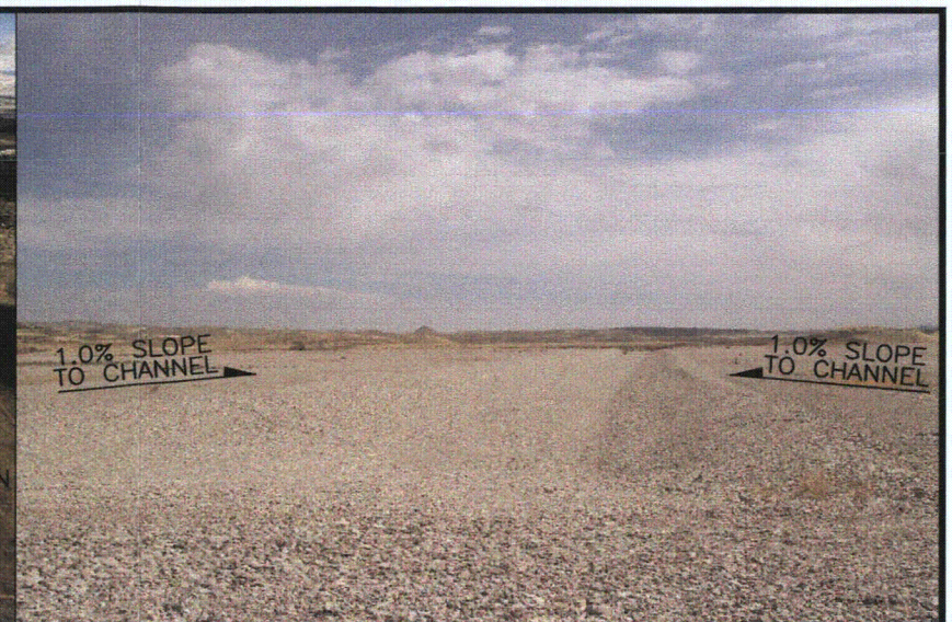
CHANNEL ON TOP OF HEAP LEACH REPOSITORY
