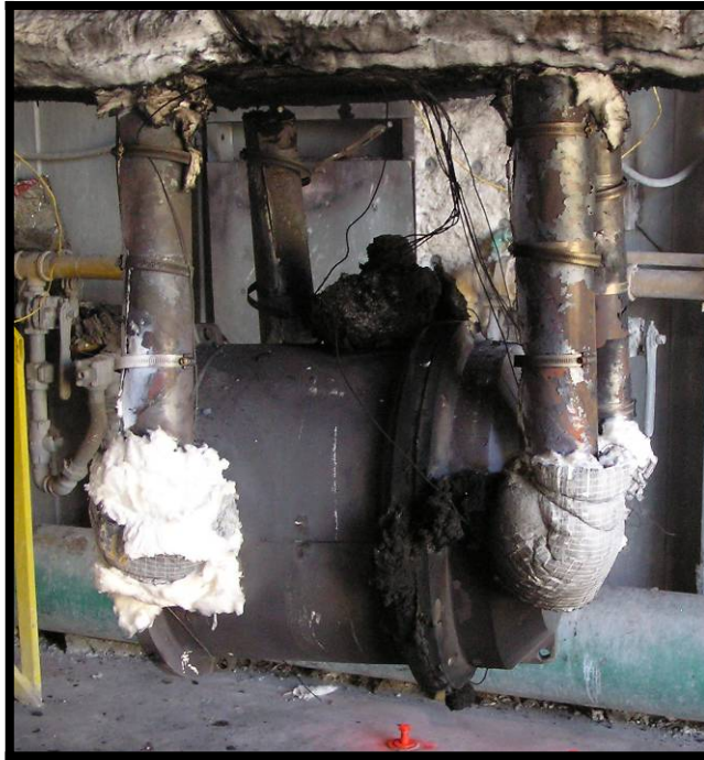
Photograph 23 – Test 2C Post-Test Condition (View 1)
