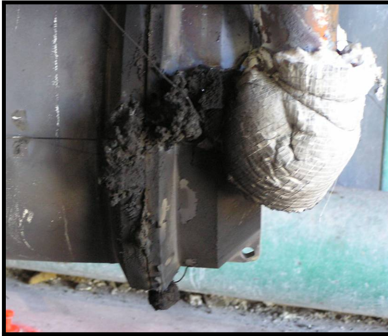
Photograph 25 – Test 2C Post-Test Condition (View 3)
