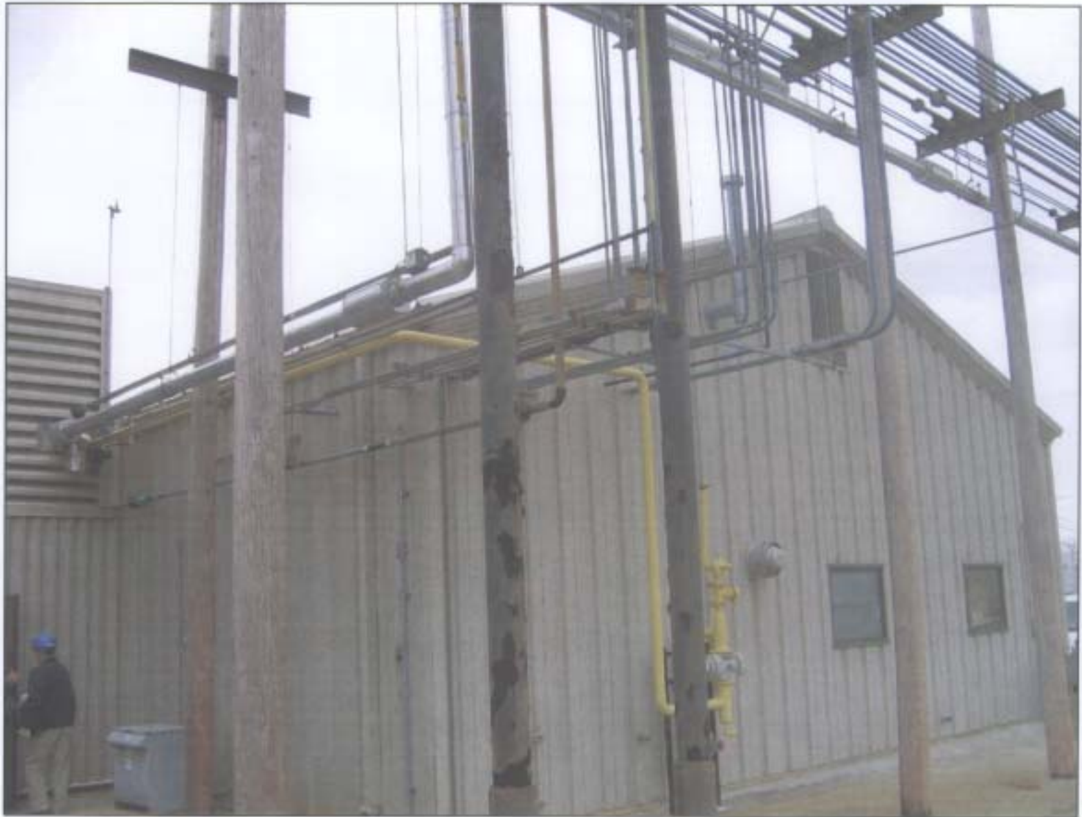
Figure 2.3 Exterior of Building 172 (Incinerator Building) Office Area
