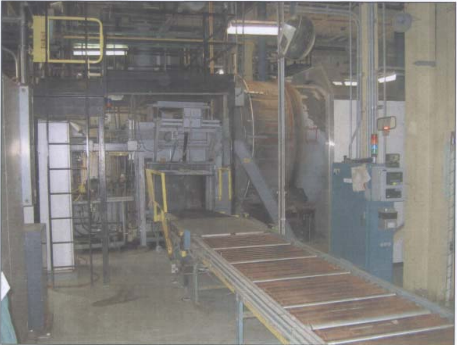
Figure 2.4 Incinerator Loading Ram and Airlock
