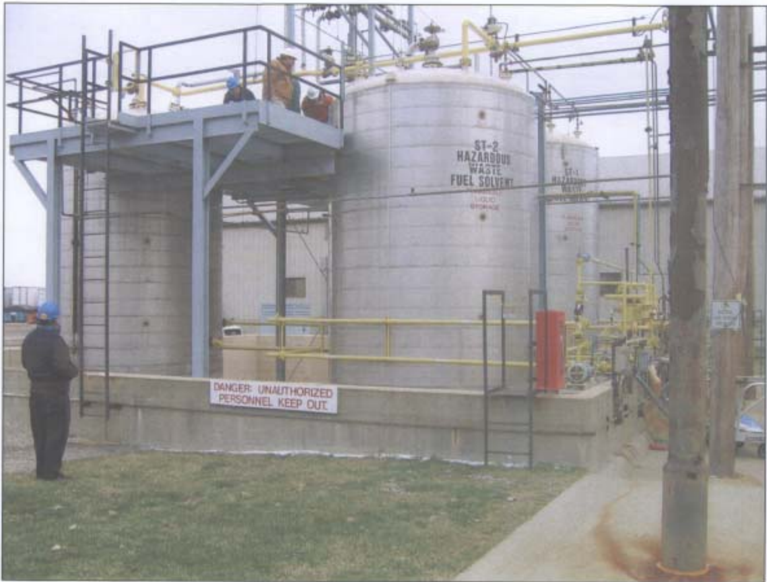
Figure 2.6 North Tank Farm
