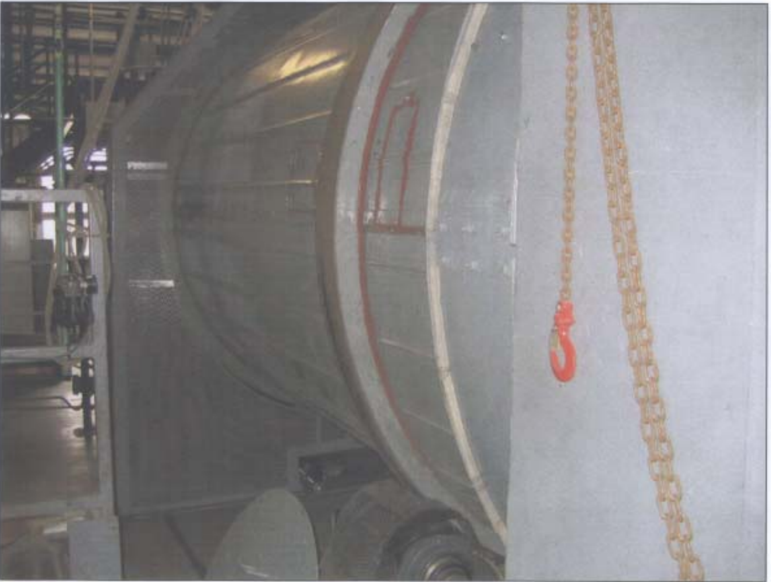
Figure 2.5 Incinerator Rotating Kiln
