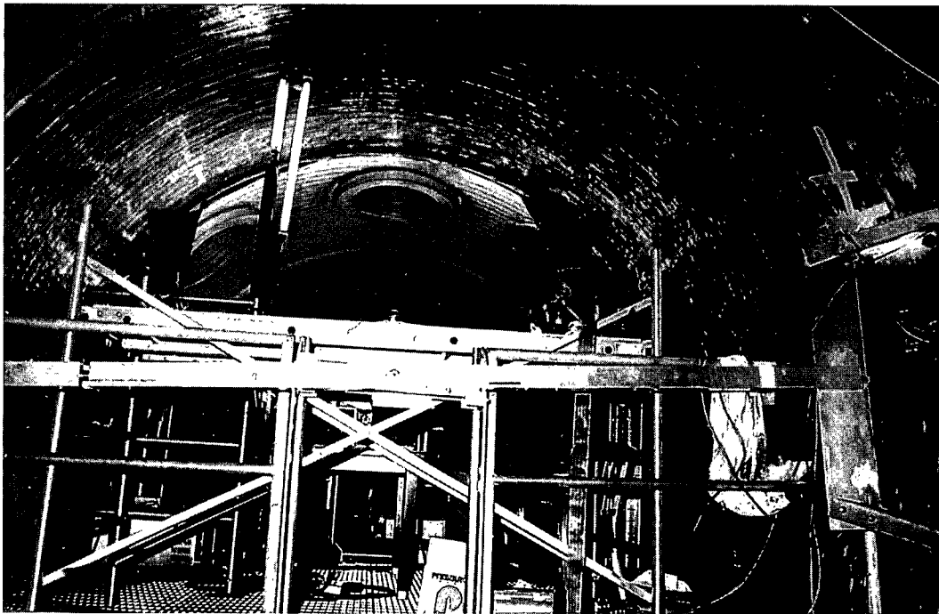
Figure 2.4 Photograph of the PVRUF vessel from the inside
