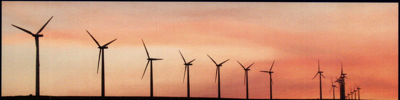
Nine Canyon Wind Project
