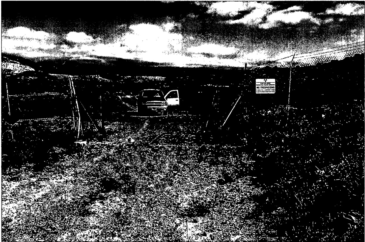
BAR 8/2006. PL-1. Damaged chain-link fence gate located in the southeast corner of the site.
