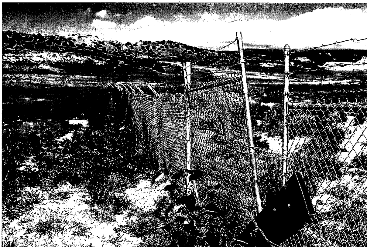
BAR 8/2006. PL-4. Poor condition of the chain-link fence in the southeast corner of the site.
