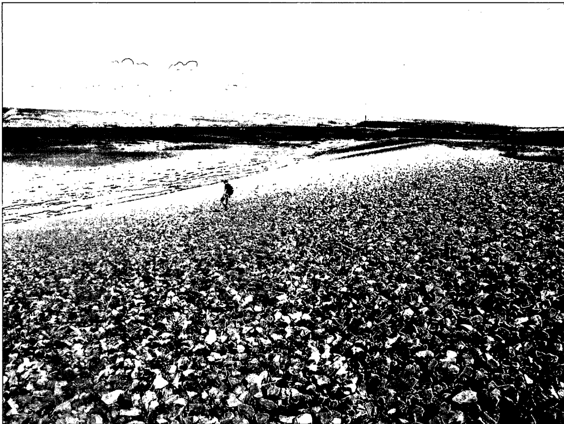
BLU 8/2006. PL-2 Southwest side slope of the main tailings disposal cell.
