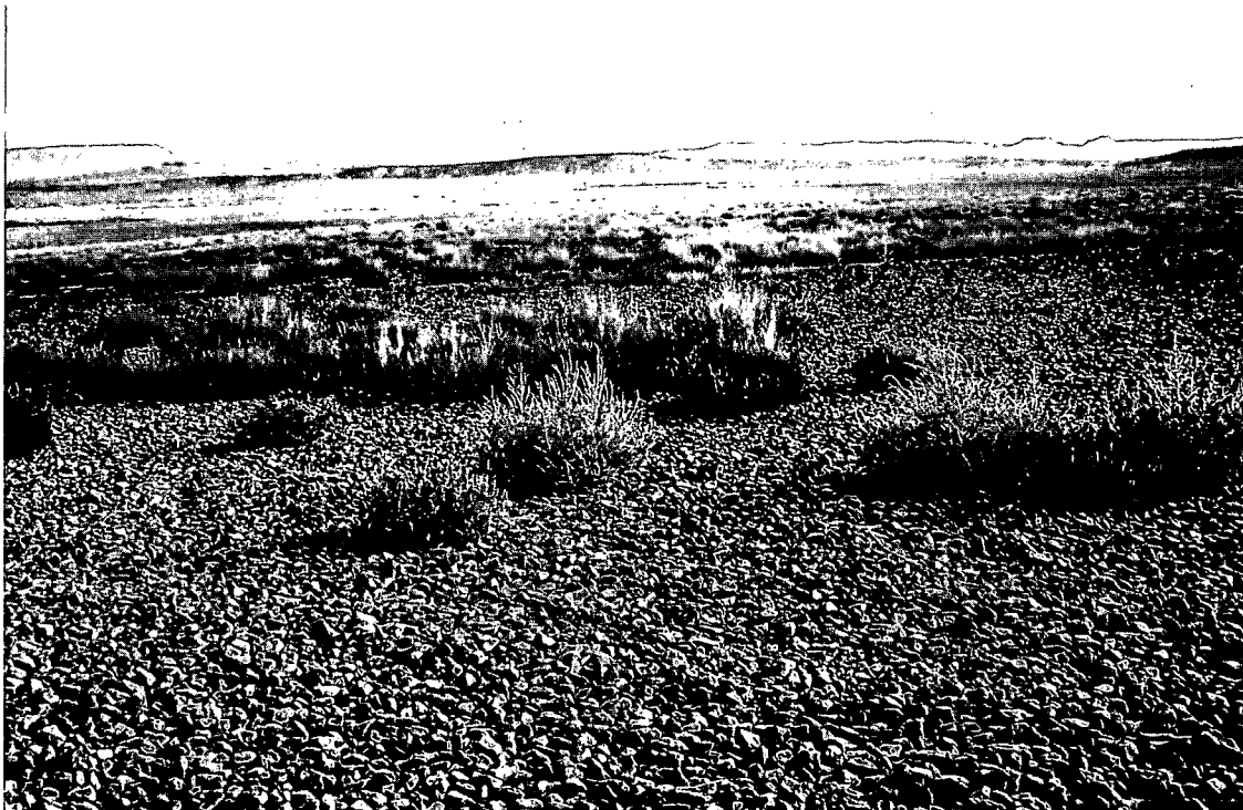
BLU 8/2006. PL-3. Top of the main tailings disposal cell viewed from the southwest corner.
