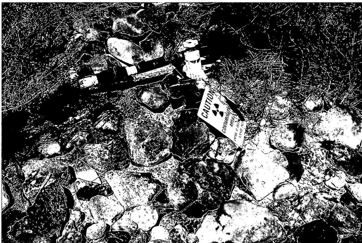
BAR 8/2006. PL-8. Contaminated drain outlet #5 at the base of the containment dam.
