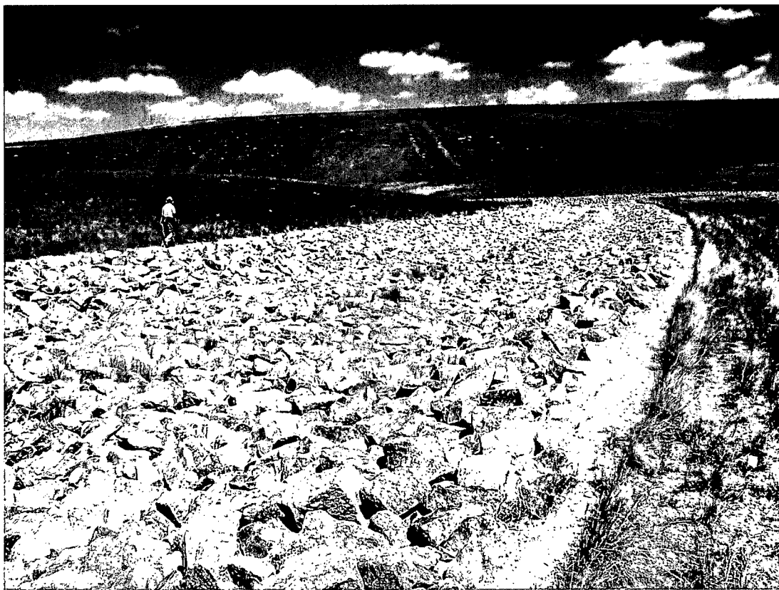
SBS 6/2006. PL-6. Riprap-armored drainage channel west of the disposal cell.
