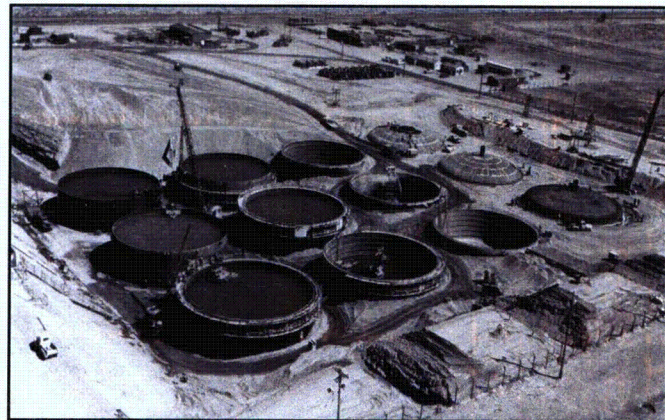
Single-Shell Tank Farm Construction – Circa 1943
