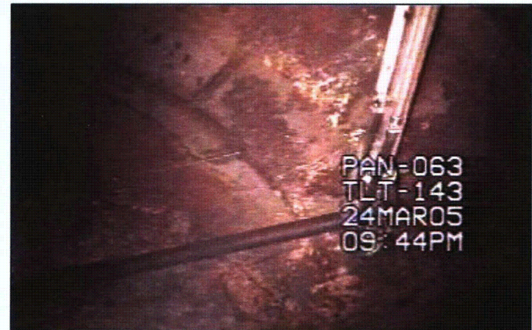
Bottom of Tank C-203 After Vacuum Retrieval
