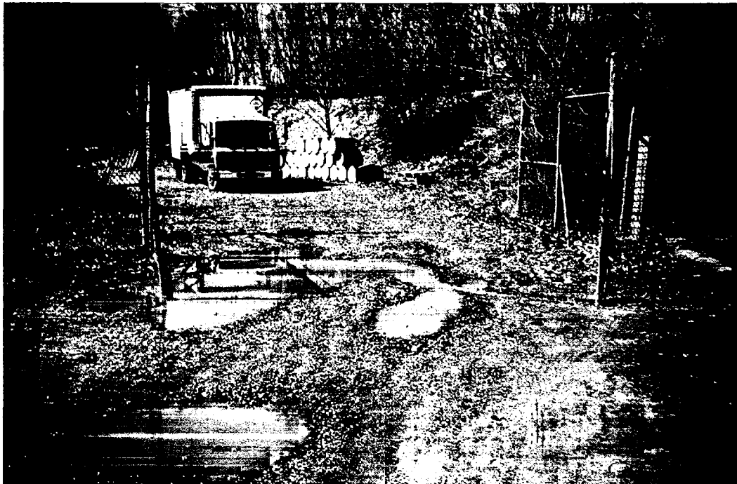
Figure 2-12 – Facility Entrance (Prior to Paving)
