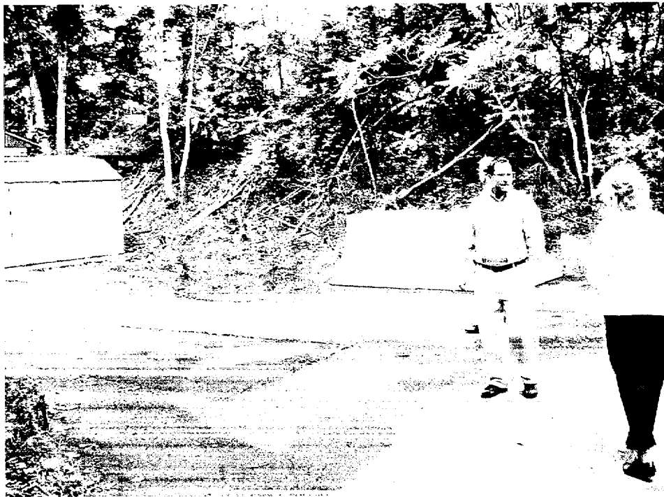
Figure 2-14 - Yard Area Looking Southwest (After Paving)
