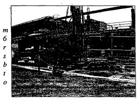
Work continues on the phase 2A onitoring wells. Pictured at left is MW-2, a 200-foot deep well located on the iverfront near the Unit 1 intake tructure. Three addition wells are eing constructed along the riverfront o help characterize groundwater flow n site.
