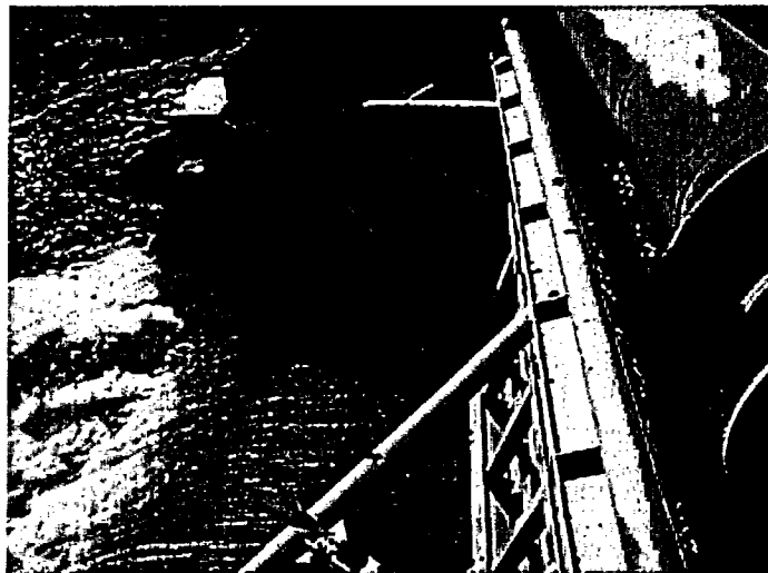
Photo No. 12 - A typical Tainter Gate. This is Gate No. 2 being operated using power from Emergency Generator. Some rust spots were noted. The Licensee's representative stated the rust spots will be painted during the 2003 maintenance season.
