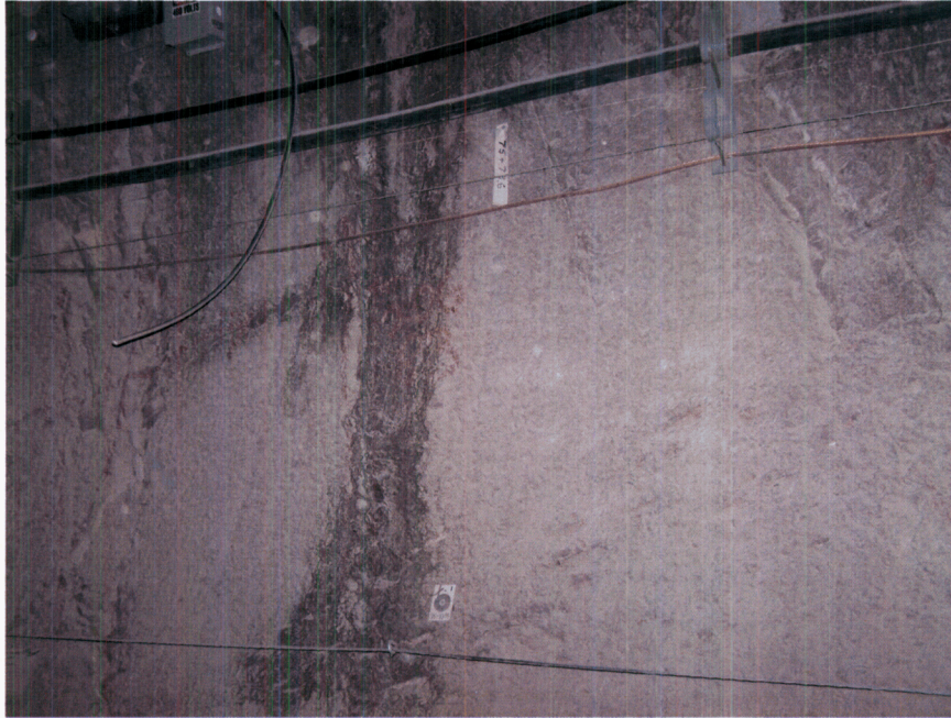
Figure 4. Photograph of Seepage Patterns on the Tunnel Walls at Exploratory Studies Facility Station 75 + 73.6 Produced by the February 2005 Seepage Event
