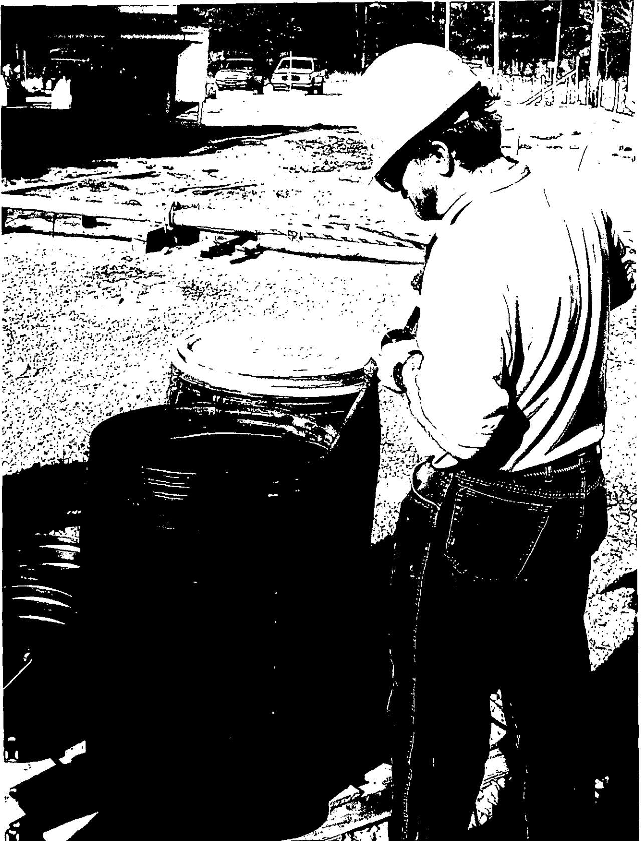
Photograph 17. The MaxFlow Air Admixture was Diluted by W. MacDonald, the Technical Representative from Celcore.
