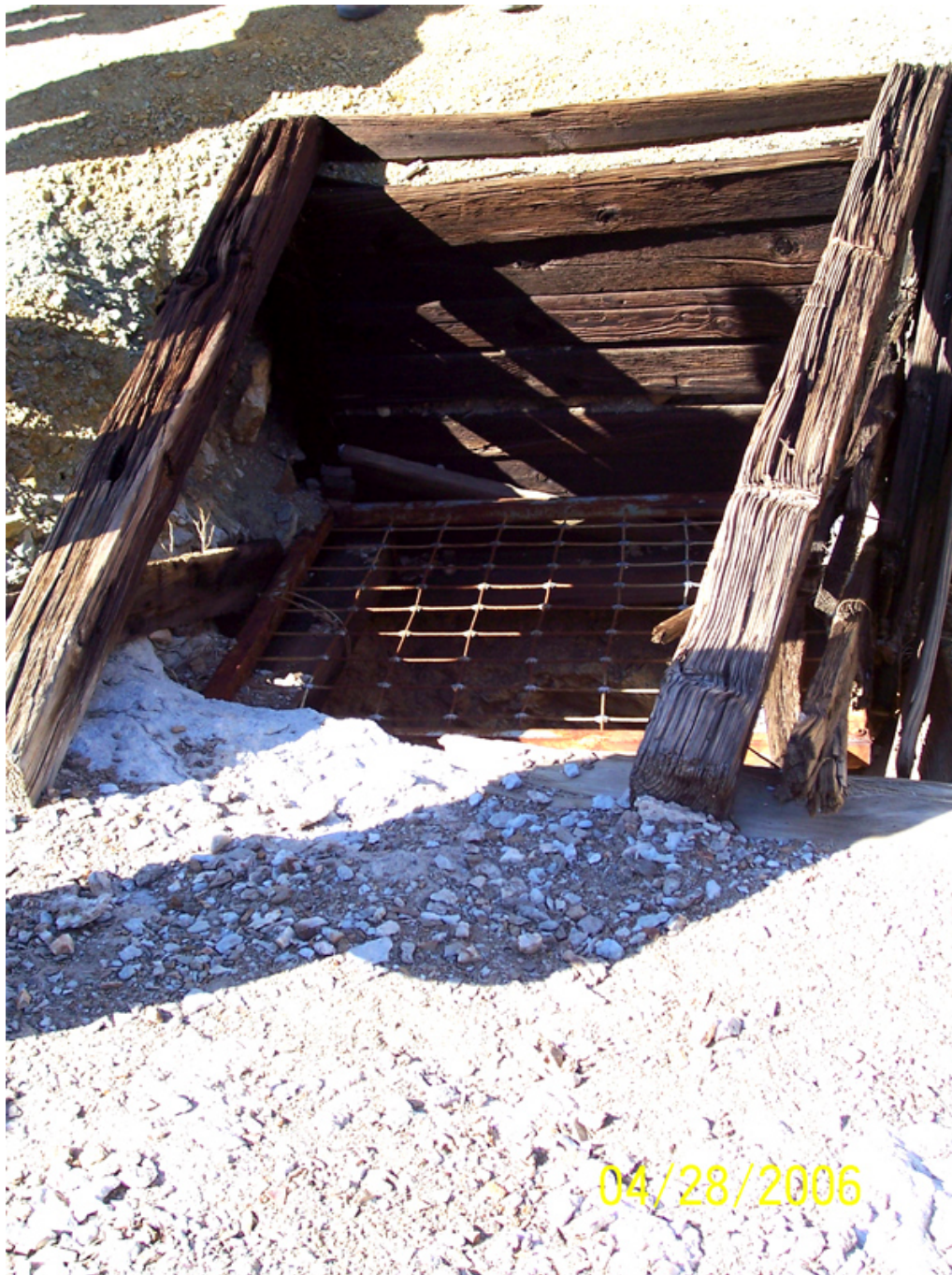
Fig. 16. Surface shaft developed by miners at Keane Wonder mine to control and capture the spring flow. Hydrogen sulfide gas was seeping from this opening.
