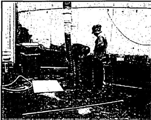
Entergy is drilling 12 new wells in the next phase of the ground water investigation. These wells are located near Unit 1 to help characterize the radioactivity associated with the Unit 1 spent fuel pool. The picture at left shows a vacuum drill being used to remove the first 5-7 feet before a drill rig with a hard tipped bit is used for the subsequent depth. Using the vacuum drill techniques helps reduce the potential to damage underground service lines.
