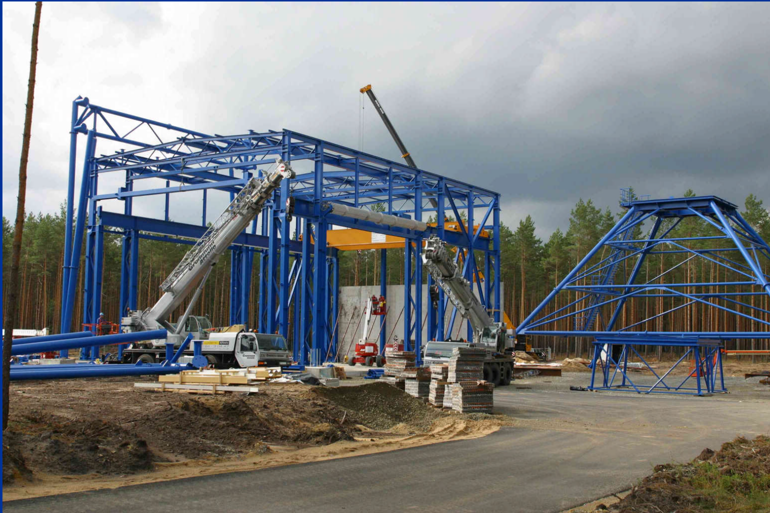
Finished skeleton of enclosed test building (left) and top of drop tower (right)
