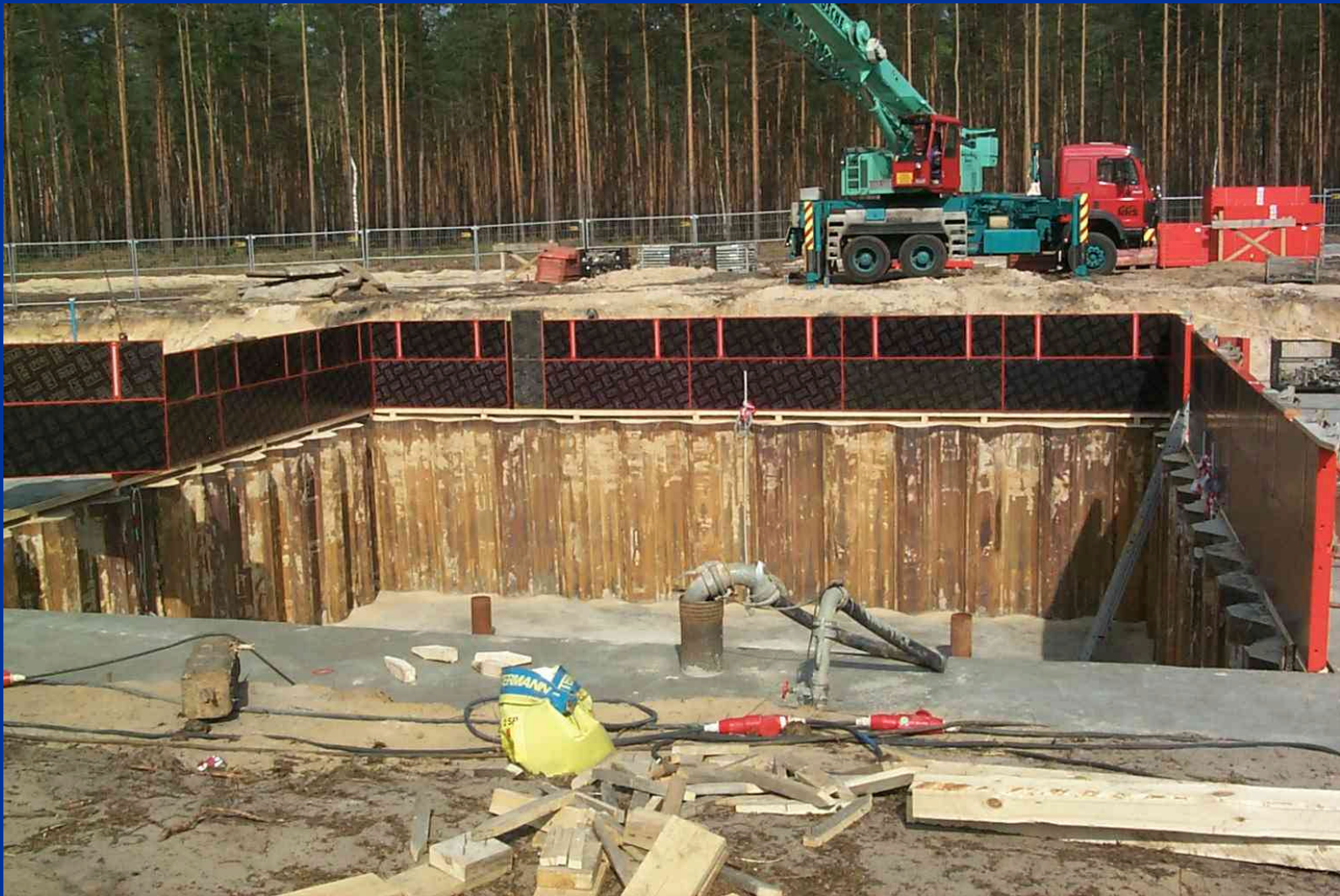
Excavation and lining of a cavity for the unyielding surface . (46 ft x 46ft x 16.5 ft).
