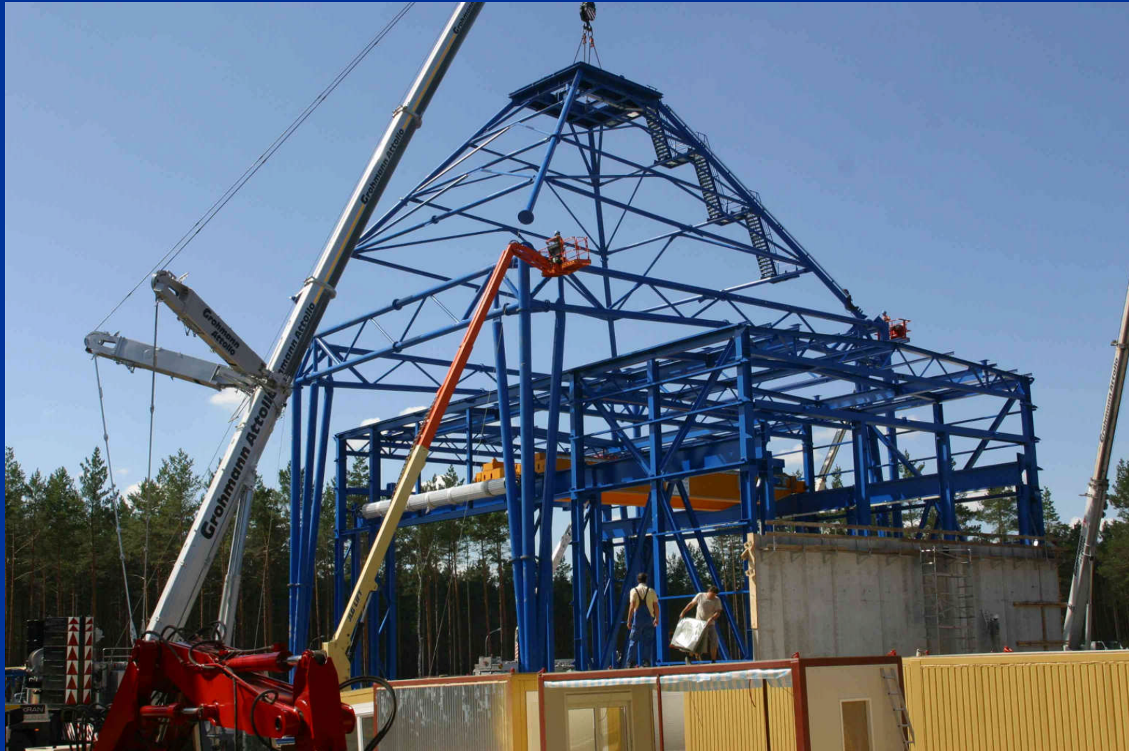
Top of drop tower being hoisted into place by an 80-ton portable crane.
