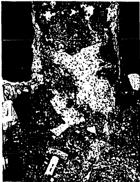
Sulfate attack of 30-year-old bridge sub-structure
