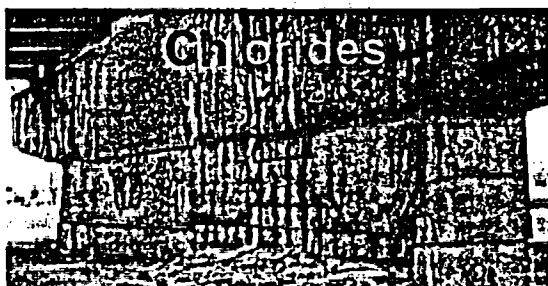
Corrosion of steel reinforcement in bridge superstructure
