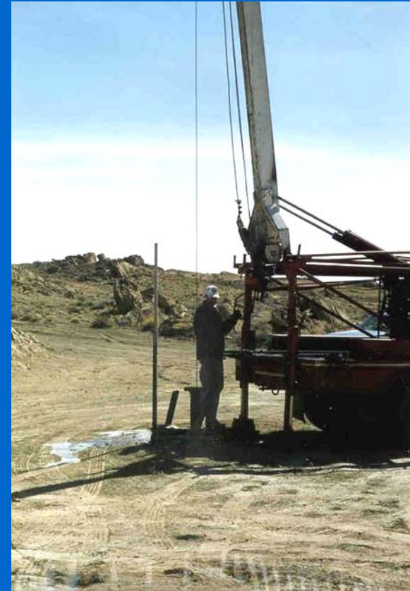
CCUCG, Purging well prior to sampling, 3/99, Monthly Inspection
