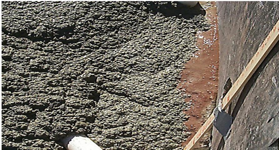
Figure RAI-17-A-5. Liquids and solids rise along the tank wall as grout is poured.
