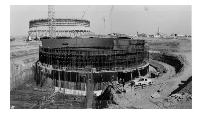
March 20, 1970 - overall view of the containment structure with cooling tower No. 1 in background
