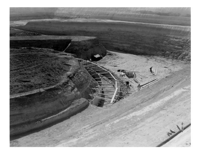
September 9, 1969 – forming for the fill concrete under the tendon access gallery floor slab
