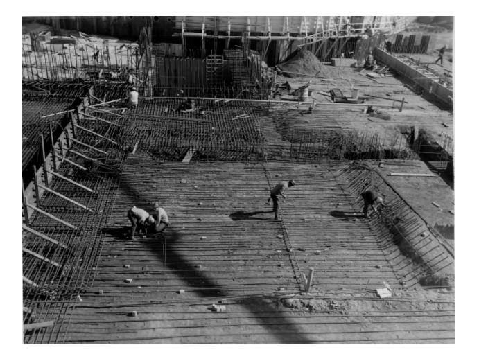
July 17, 1970 – auxiliary building showing reinforcing being placed
