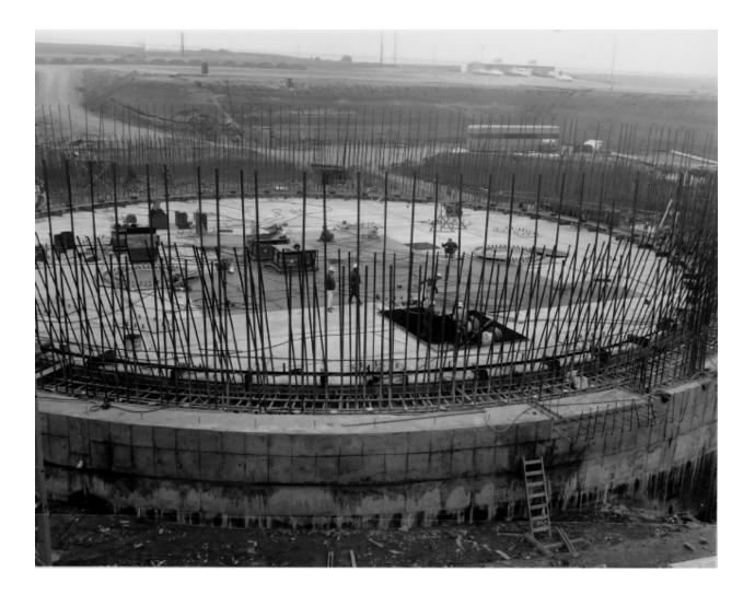
February 9, 1970 – installing floor liner plate on reactor building floor slab
