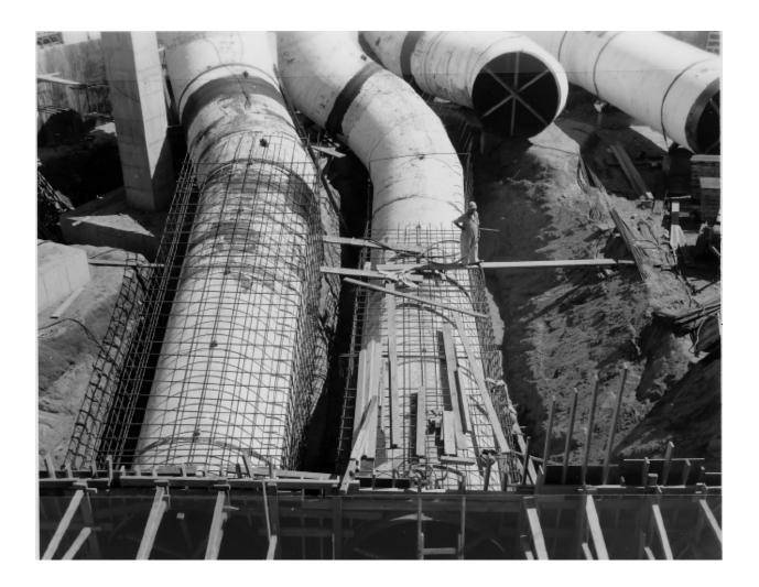
April 24, 1970 – 108" diameter circulating water pipe forming and reinforcement for concrete encasements
