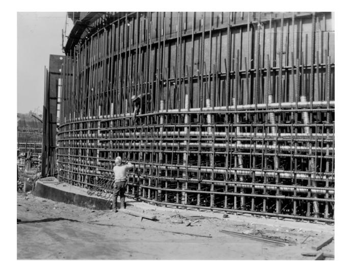
April 23, 1970 - reinforcing steel and tendon sheathing for the first lift of the containment wall
