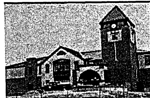
New school under construction.
