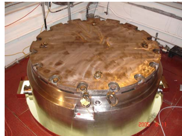
Cask Cover Installed
