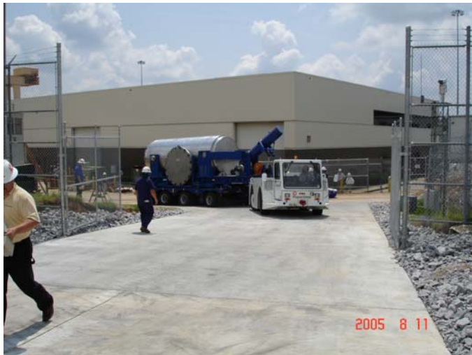
Driving Up New Heavy Haul Path
