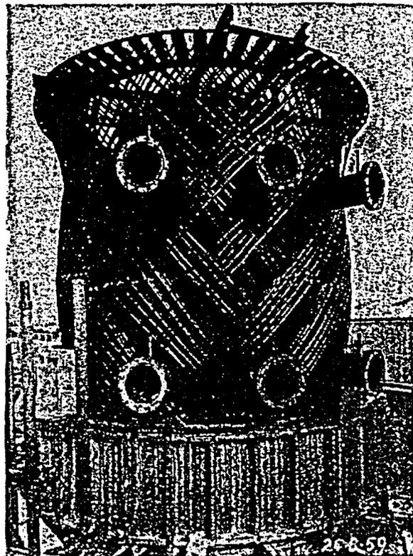
**Figure 149** 1:8-scale cylindrical PCRV model. Source: D. C. Price and M. S. Hinley, "Testing a 1/8th Scale Cylindrical Vessel," Group G, Paper 43, *Prestressed Concrete Pressure Vessels*, Institution of Civil Engineers, London, pp. 489–496, 1968.
