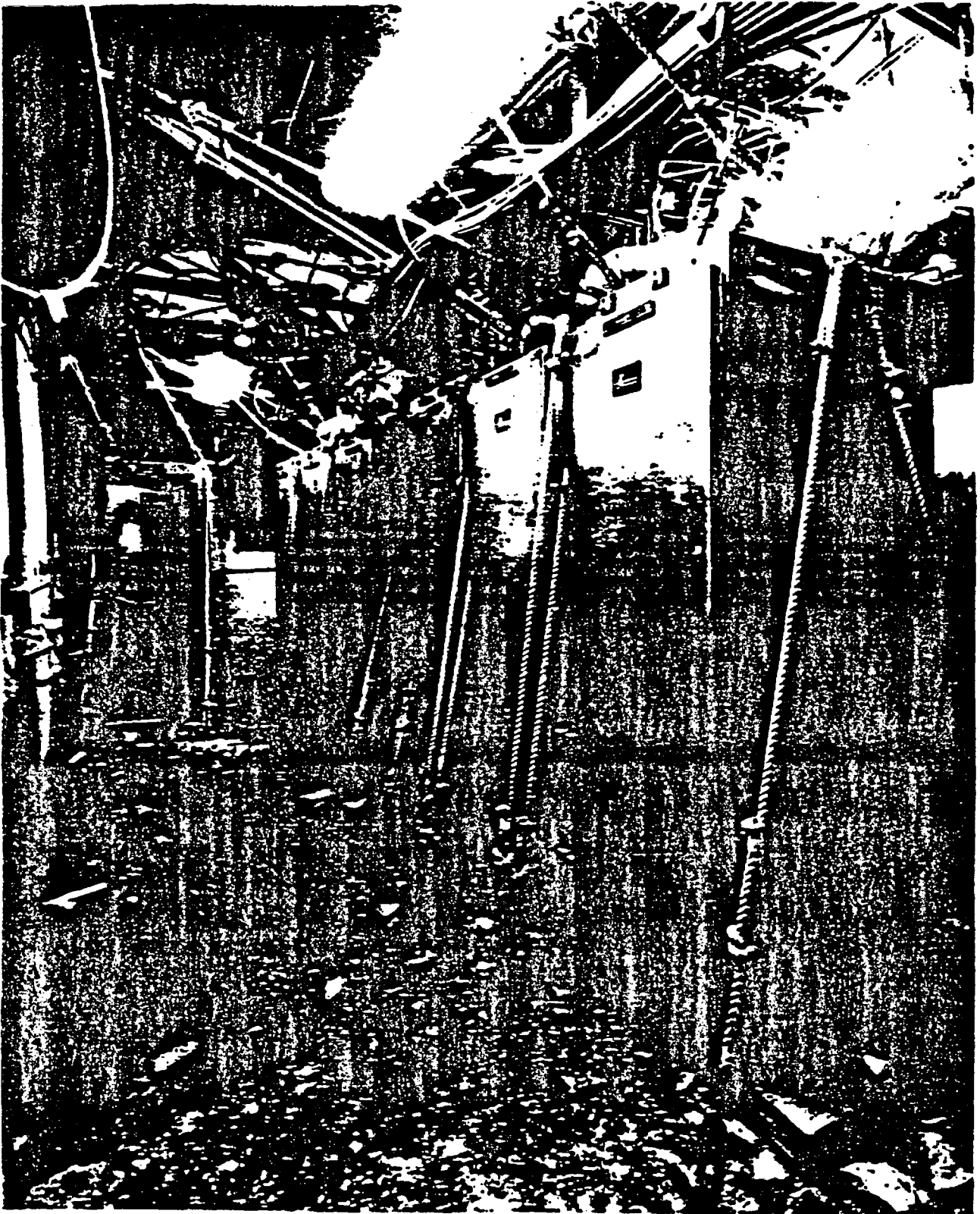
Figure 42 — Previous Tunnel Event Postshot Damage, HURON LANDING Instrumentation Alcove
