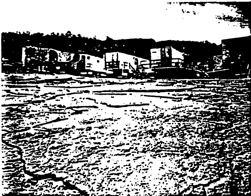
PHOTO F. — Non-subsidence-related cracks on the MILAGRO pad. View looking west.
