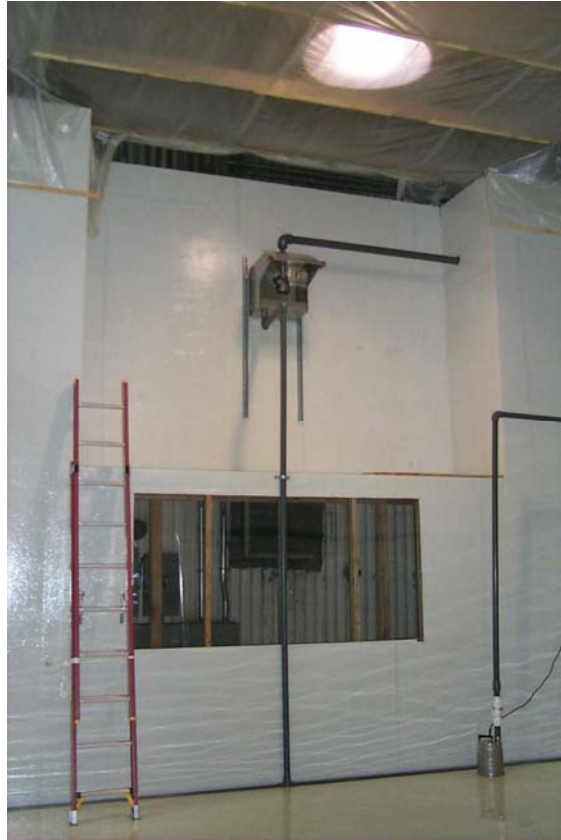
Figure 9. Wash ball mounted in mockup structure prior to washing.
