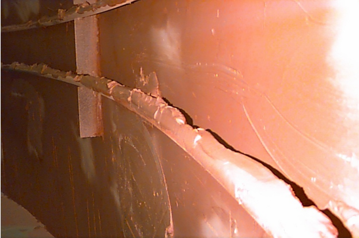
Figure 13. Mockup tank wall cooling coils covered with surrogate solids.
