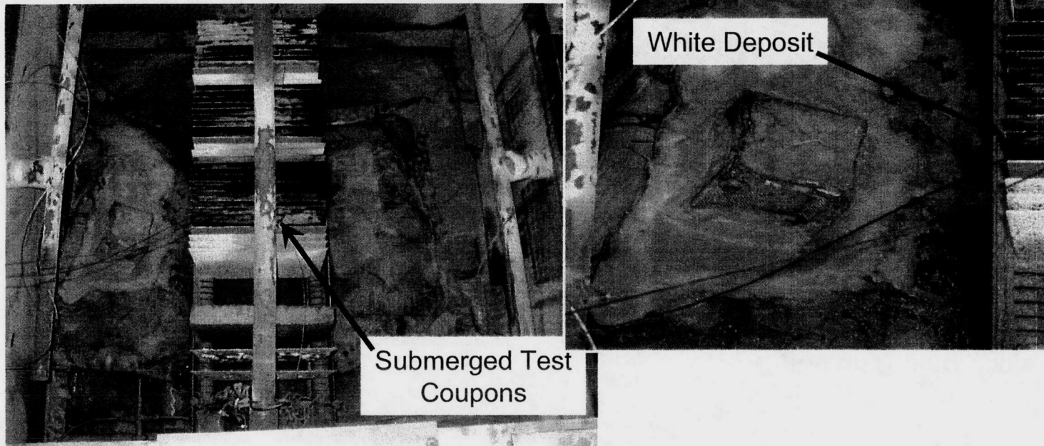
Test Chamber: Top View after Draining
