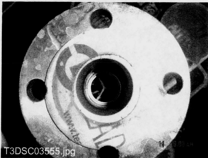
CalSil on Flowmeter Struts
