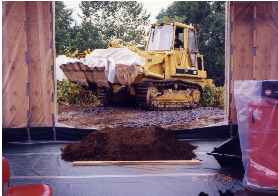
Photograph 20 Quarry Area Soil Processing September 27, 1996
