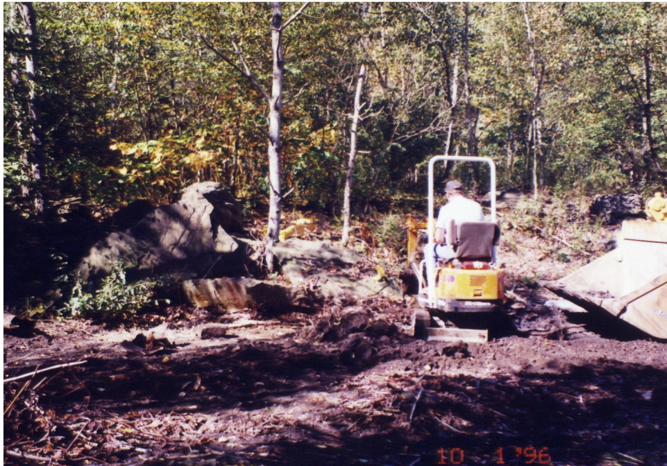
Photograph 27 Quarry Area Remediation October 1, 1996
