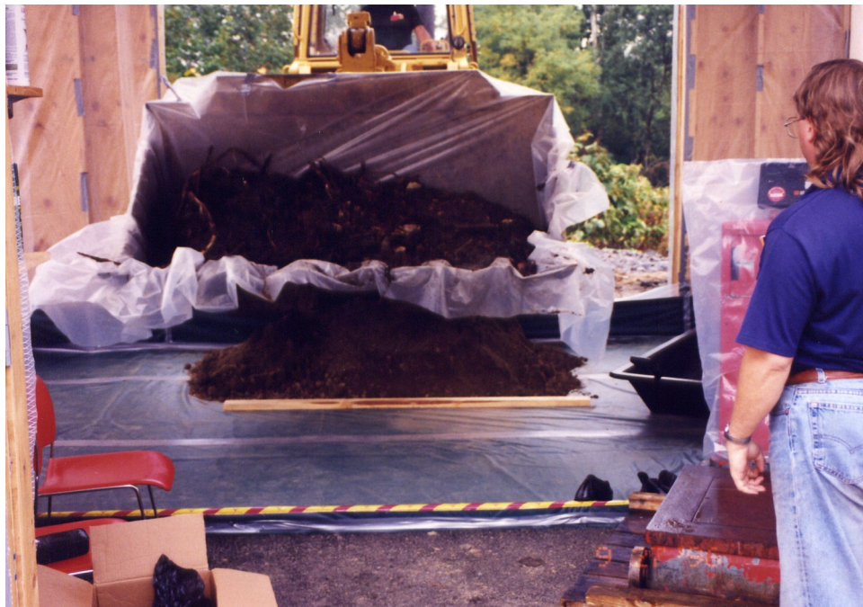
Photograph 21 Quarry Area Soil Processing September 27, 1996
