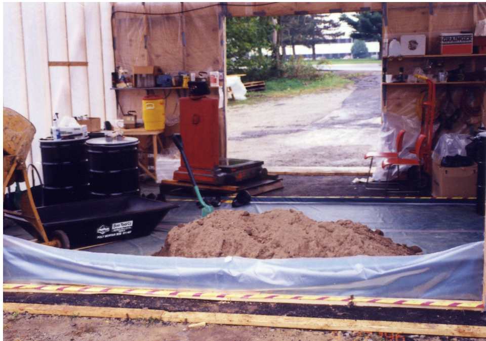
Photograph 18 Quarry Area Soil Processing September 27, 1996
