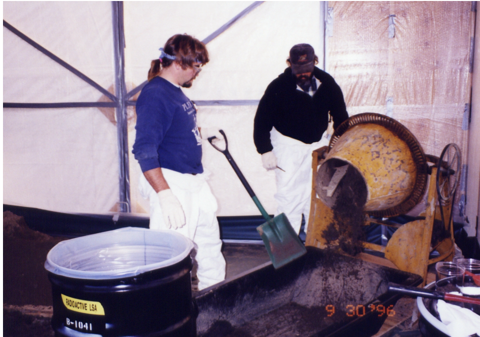
Photograph 22 Quarry Area Soil Processing September 30, 1996
