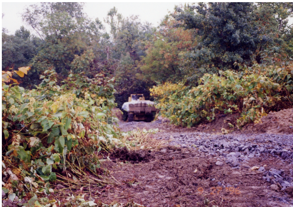
Photograph 19 Quarry Area Soil Processing September 27, 1996
