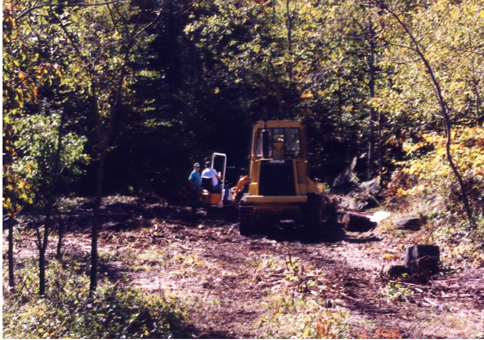
Photograph 26 Quarry Area Remediation October 1, 1996
