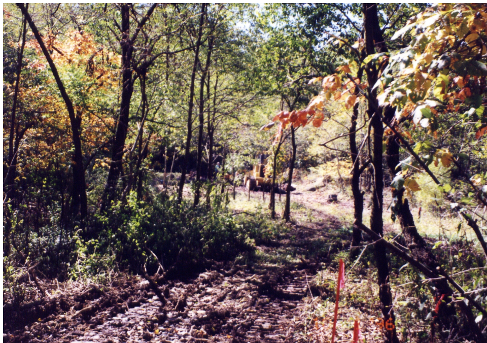
Photograph 25 Quarry Area Remediation October 1, 1996
