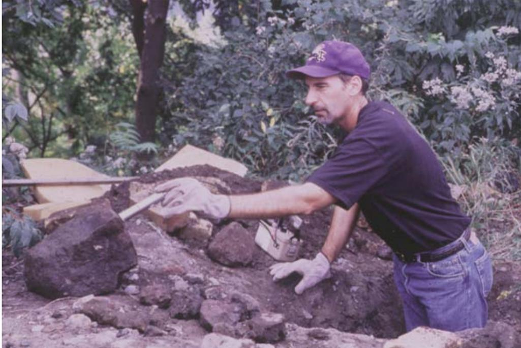
Figure 1-1. Sites B and C were covered with approximately 0.3 to 1.0 m of soil and construction debris. At Site B a small pit was excavated on top of the site to collect slag samples. The large block being pointed to had a prominent brownish weathering rind visible on the right side of the block.
