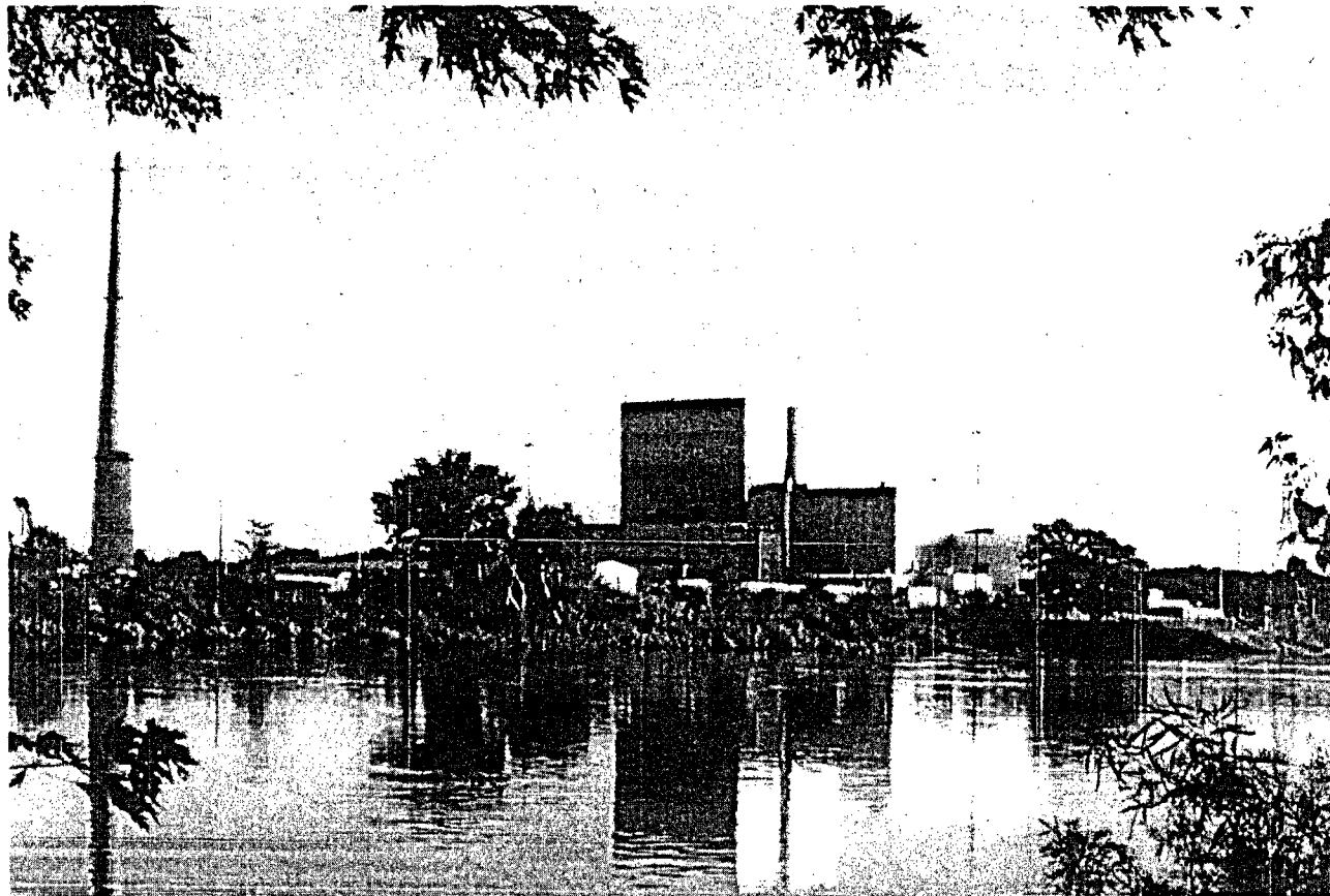
Monticello Nuclear Generating Plant
