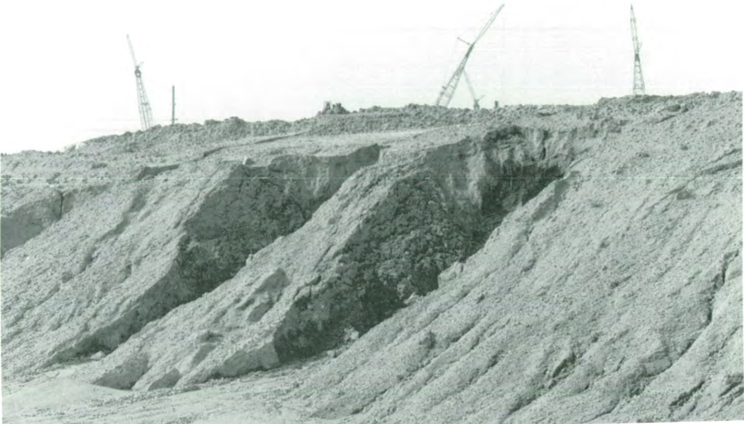
Figure 3.—Erosion on unstabilized banks in an area of Udorthents, friable substratum.
