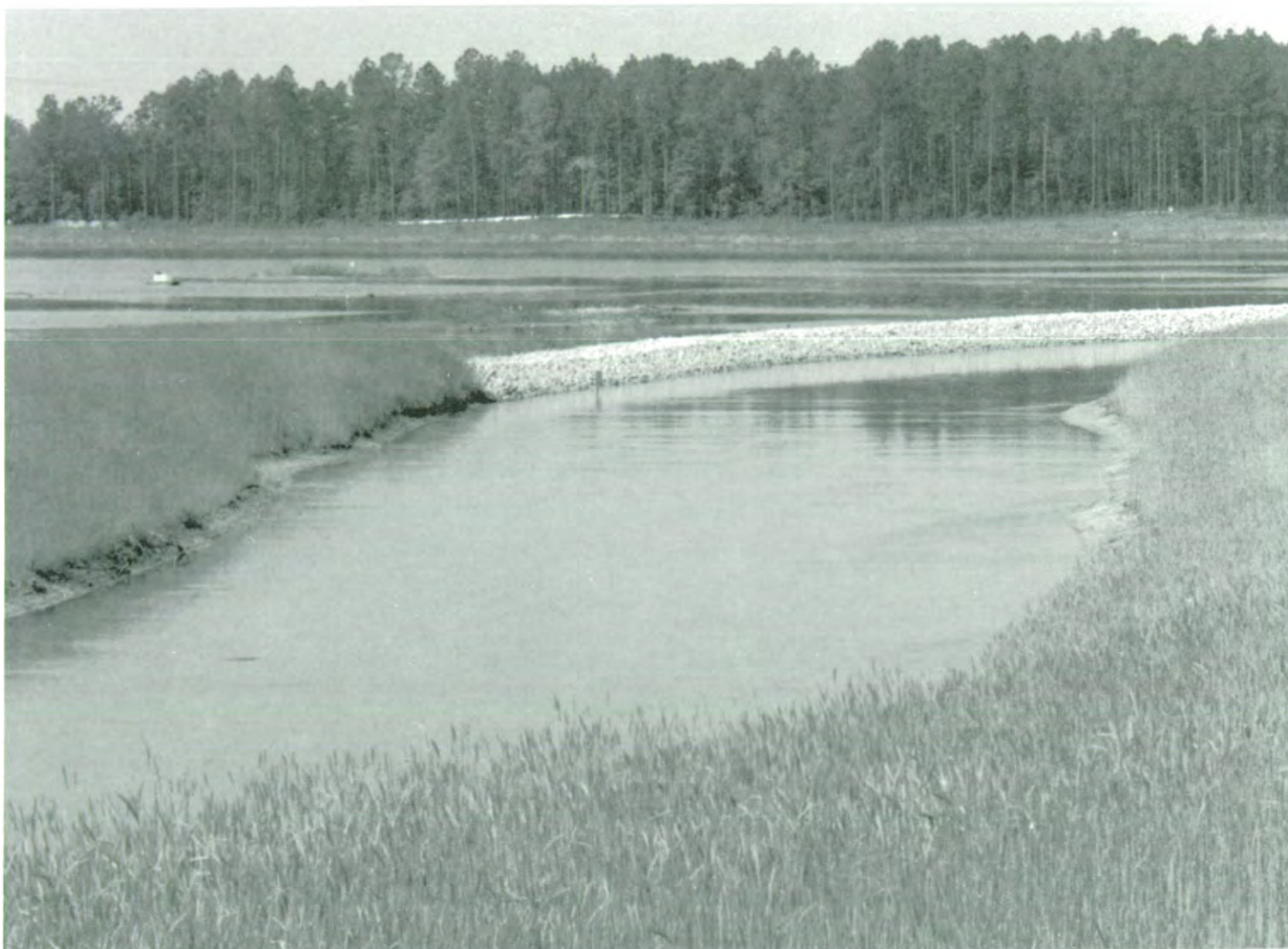
Figure 7.—A properly designed cooling pond with shaped and vegetated banks, which help to control erosion.
