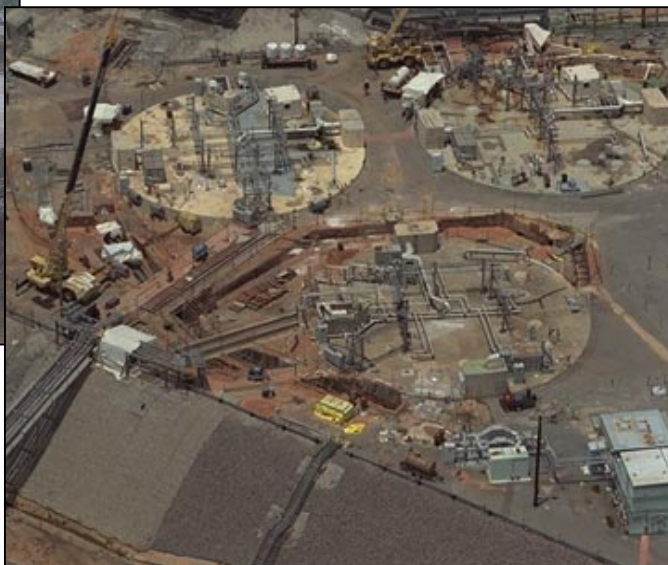
Overhead View of H Tank Farm showing the tops of three tanks. Each tank is approximately 90 feet across and can contain over one million gallons of waste.
