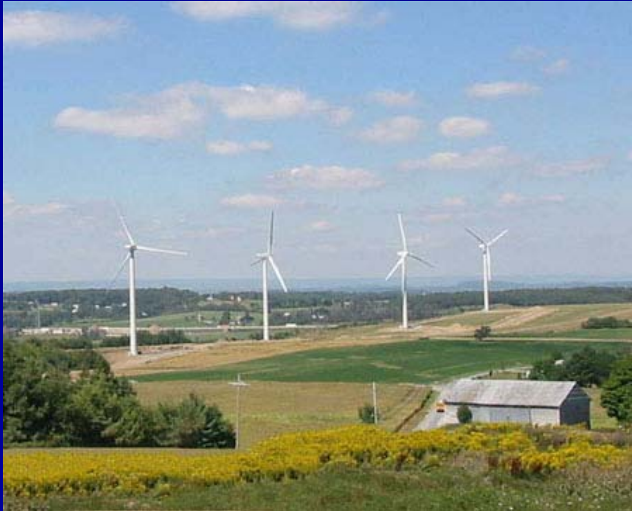
Somerset Windfarm, Pennsylvania
