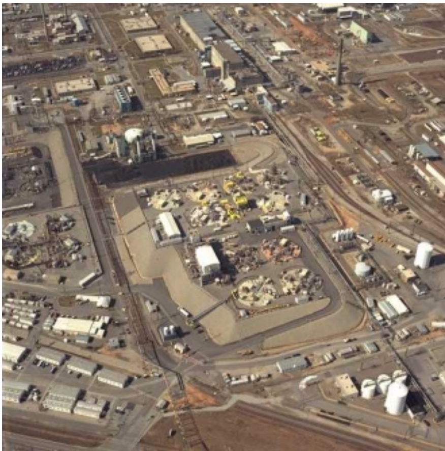
Twenty-nine underground storage tanks are located in SRS's H-Area Tank Farm. The tanks, built of carbon steel inside reinforced concrete containment vaults, hold high-level liquid radioactive waste. Twenty similar tanks are located in the site's F-Area Tank Farm.
