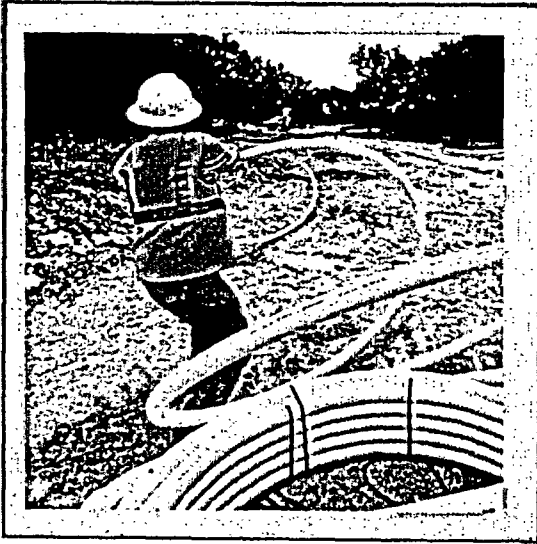
Reynaldo Carabajal, Construction and Maintenance Technician, uncoils piping at a construction site in New Braunfels, Texas.
