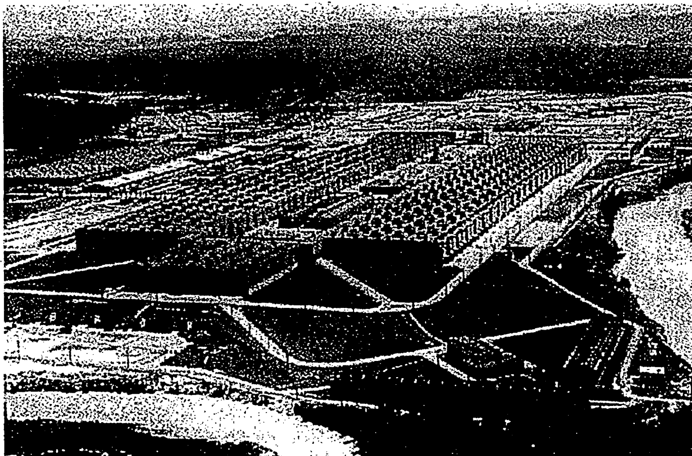
Figure 2: Oak Ridge gaseous diffusion plant, built during World War II. At the time of its construction this was the largest industrial building in the world. In part it was decided to locate this plant in Tennessee so that its large electricity demand could be met by the abundant coal and hydroelectric plants built by the government run Tennessee Valley Authority. It is now closed and awaiting decommissioning. (photo taken from the website of the "Scientific History of the Atomic Bomb" online at http://www.hcc.mnscu.edu/programs/dept/chem/abomb/K25_Aerial.jpg )
