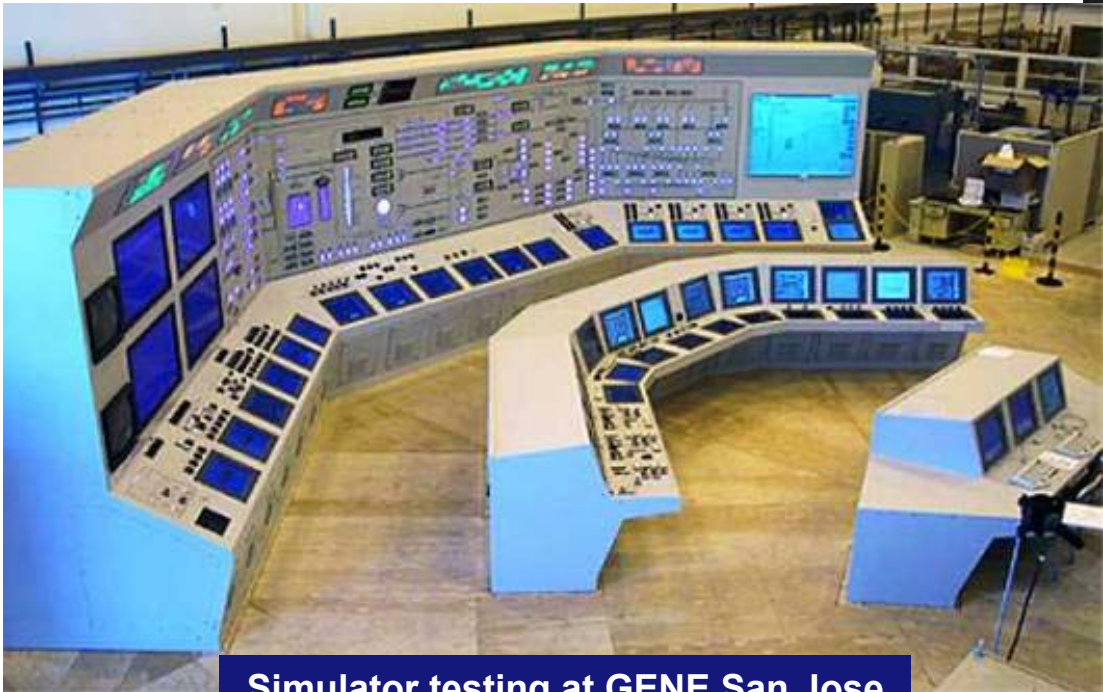
Main Control Room Panels Testing
