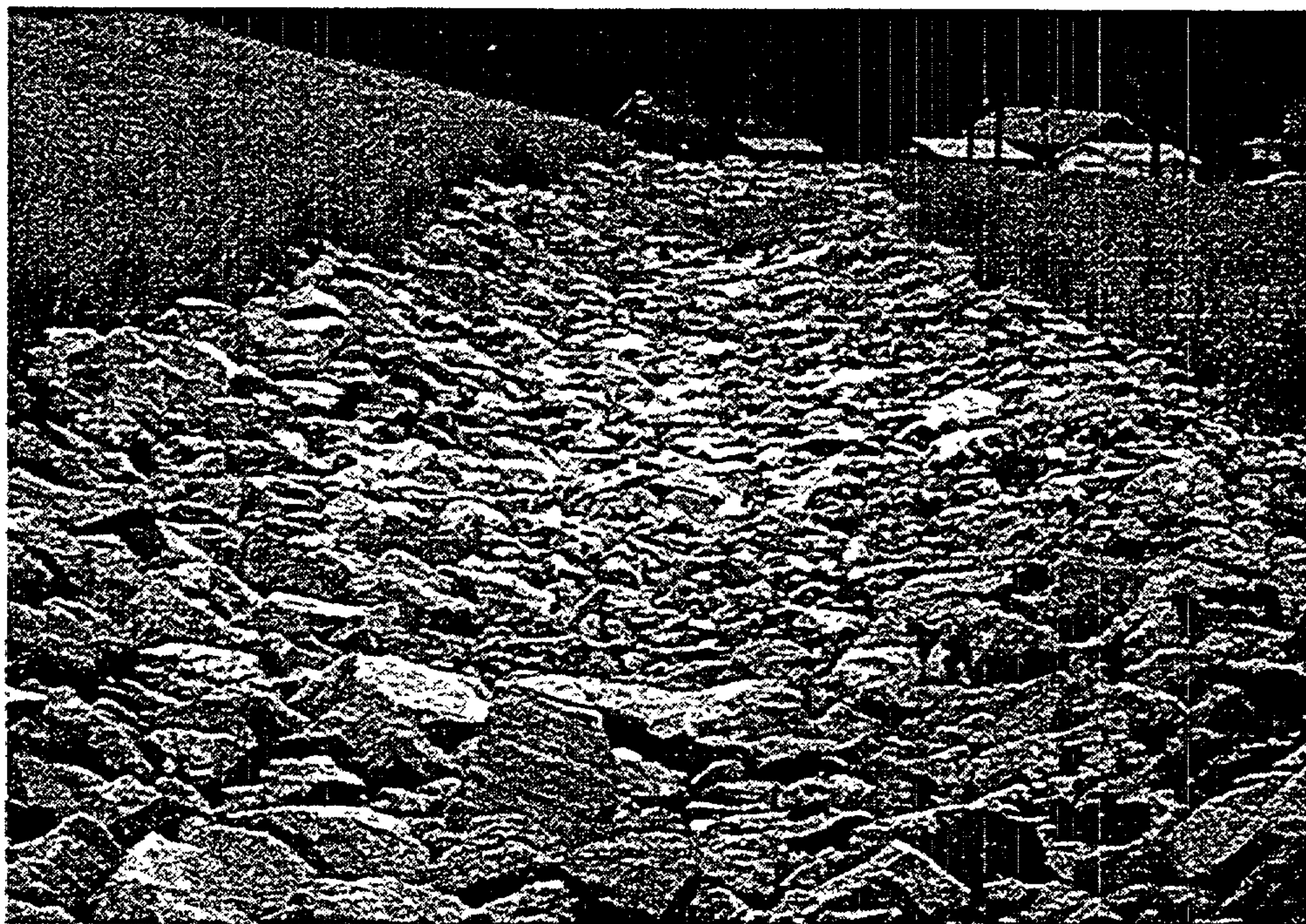
Figure F-2. Marginally-placed riprap
