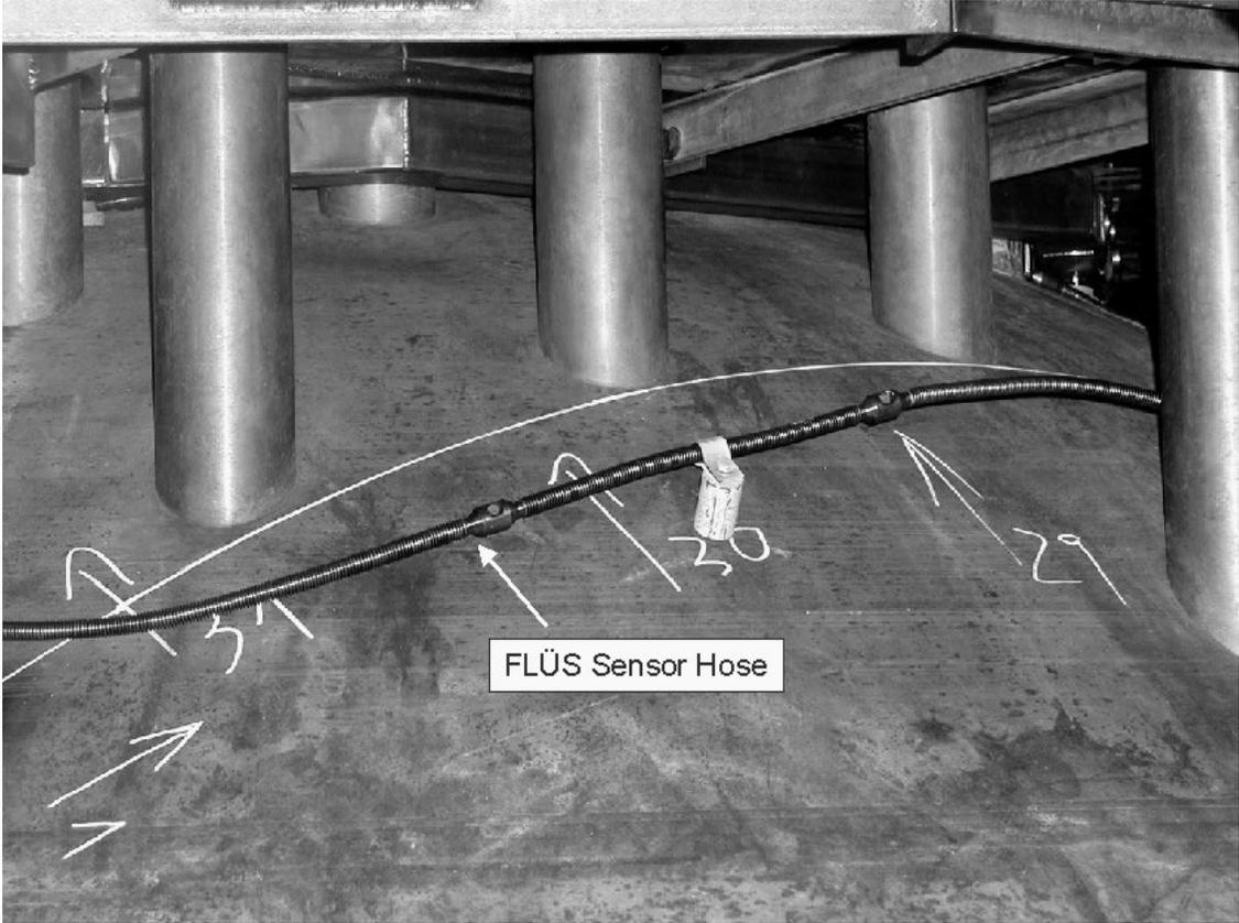
Figure 5 FLÜS Sensor Hose installed on RPV head of KWO
