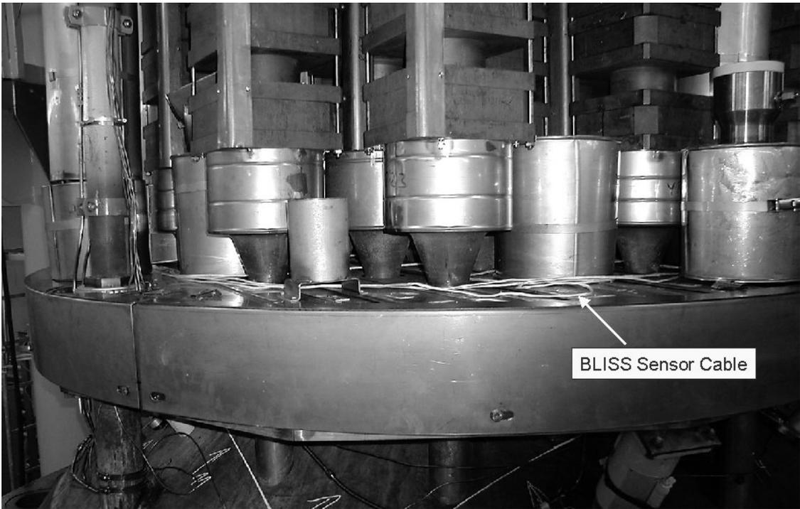
Figure 4 BLISS Sensor Cable installed on RPV Head
