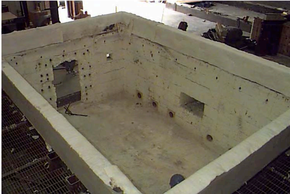
12' x 18' Horizontal Furnace (Overhead View)
