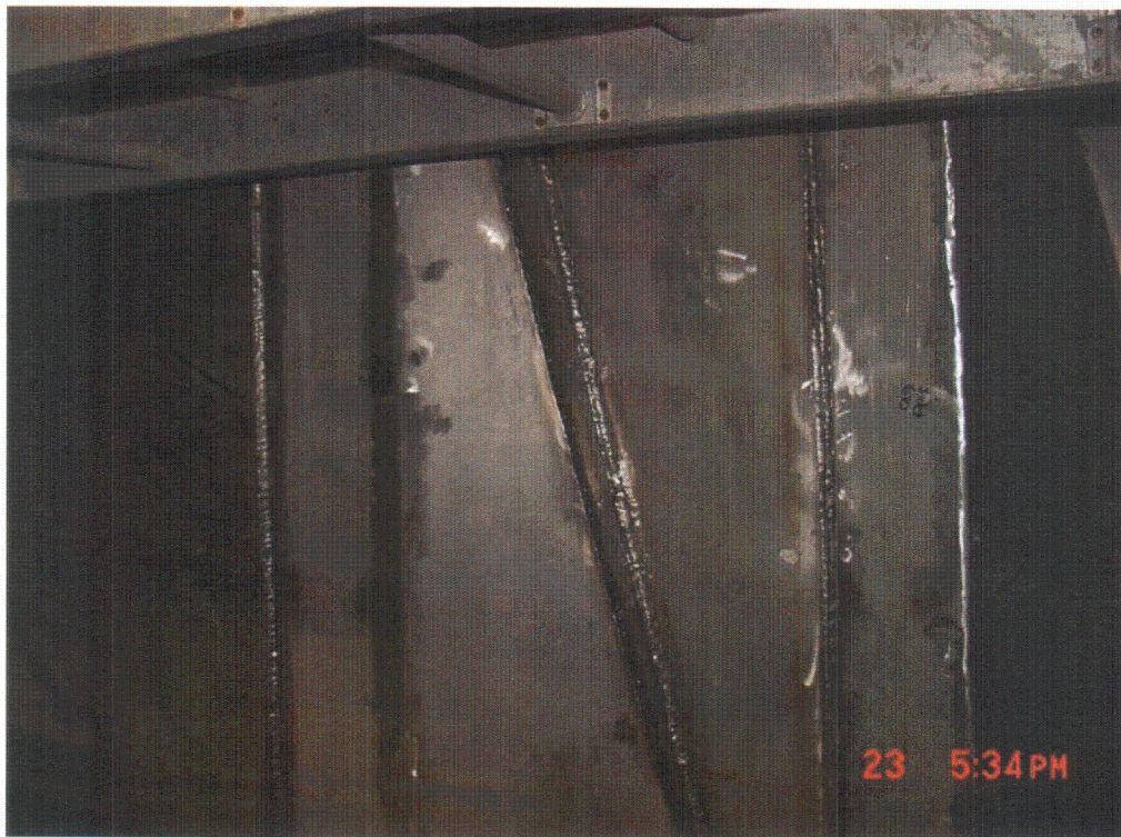
Figure 31: Response locations on upper right part of 0 degree side of dryer #1.
