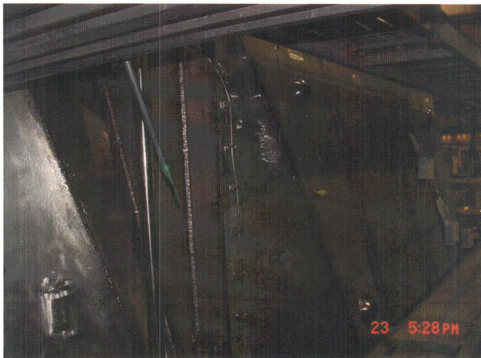
Figure 18: Full view of 270 degree hood of dryer #1 (before installation of temporary sensors).
