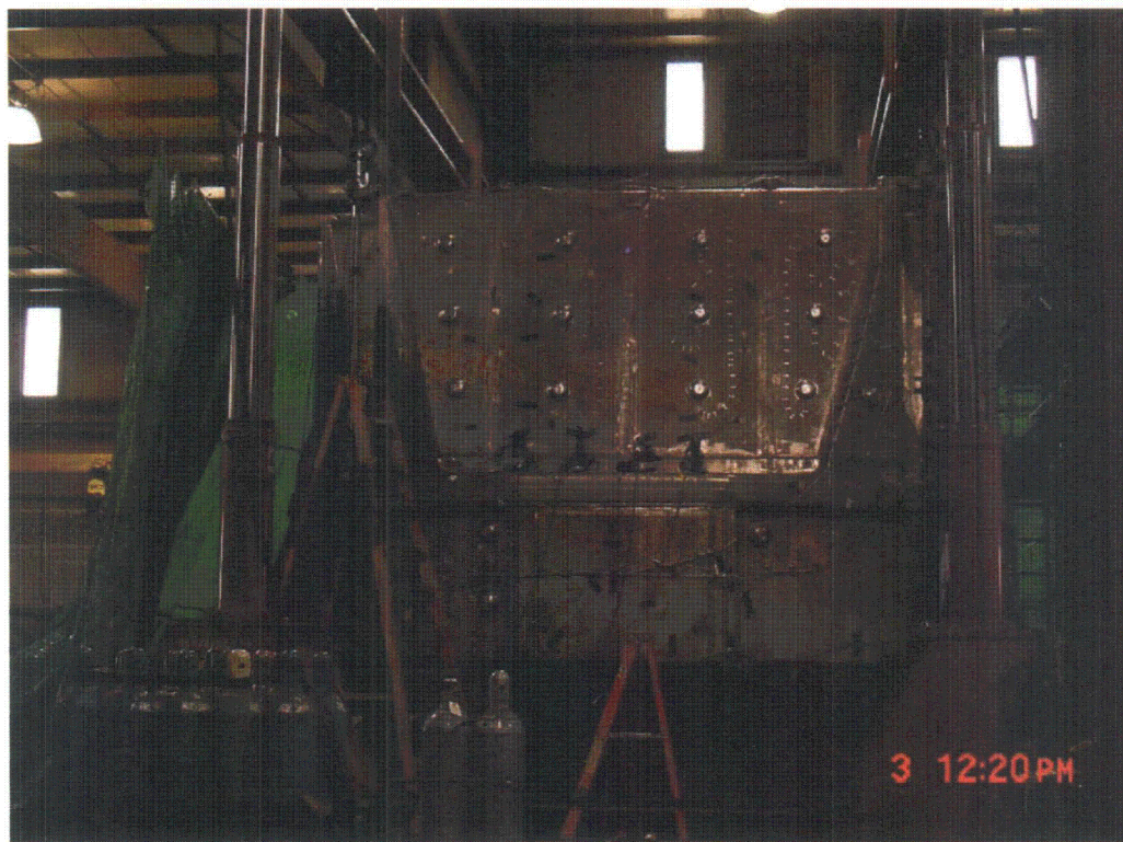
Figure 9: Full view of 90 degree hood of dryer #1 during measurements.
