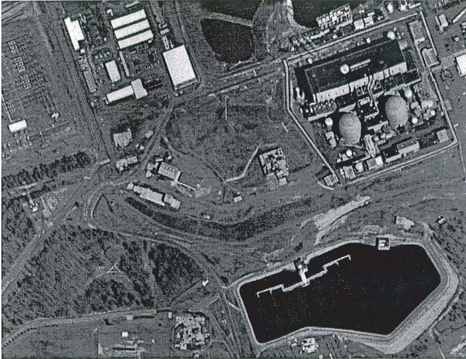
Figure 2.5-66 Photograph of Plan View of Slope North of the SWR
