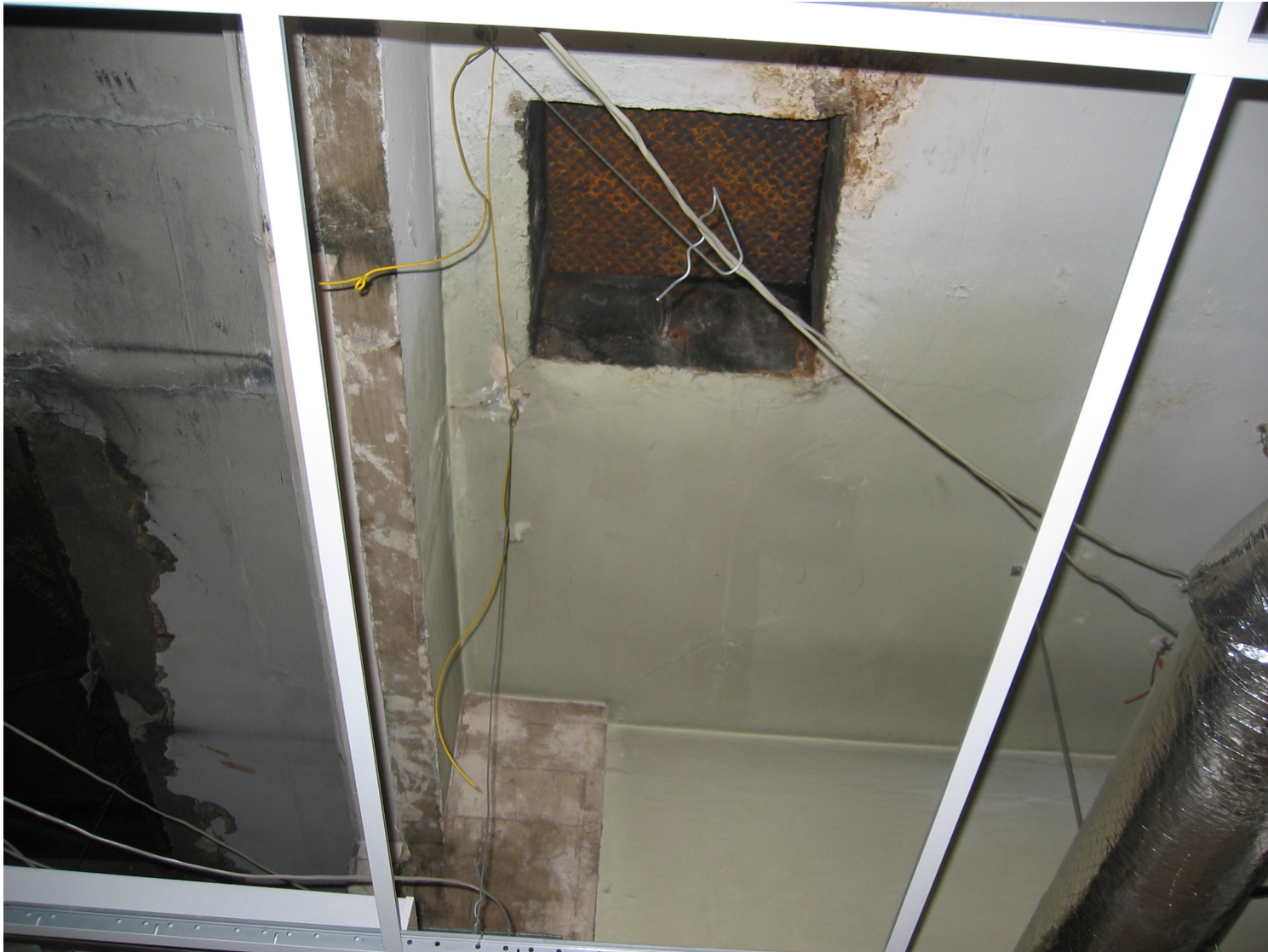
Closer detail of hood duct chase
